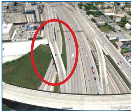
Braided ramps in the Marquette Interchange
