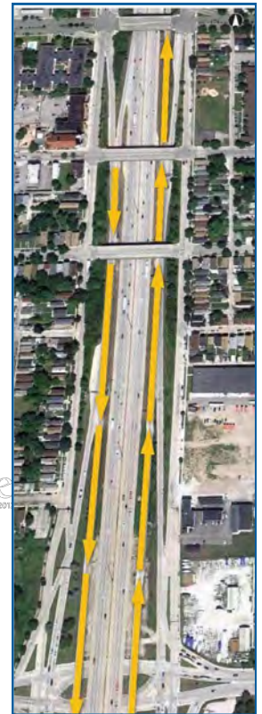
Collector-distributor road I-43/I-94 at Becher St.
