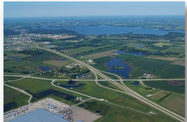
County A Interchange
