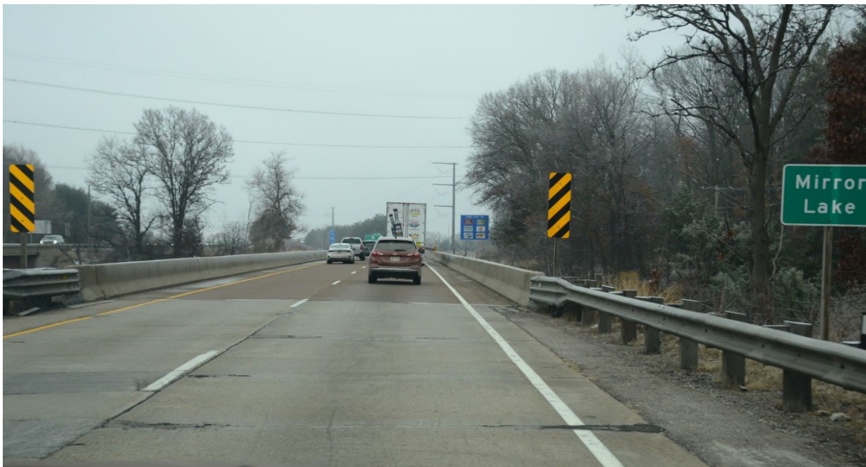
Figure 6. I-90/I-94 Approaching Mirror Lake Bridge, Southbound
