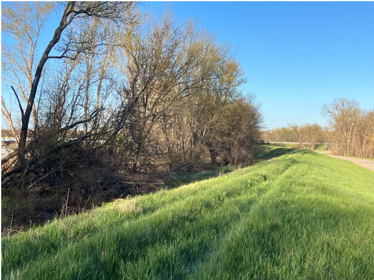
Figure 2-1: Existing Caledonia Levee
