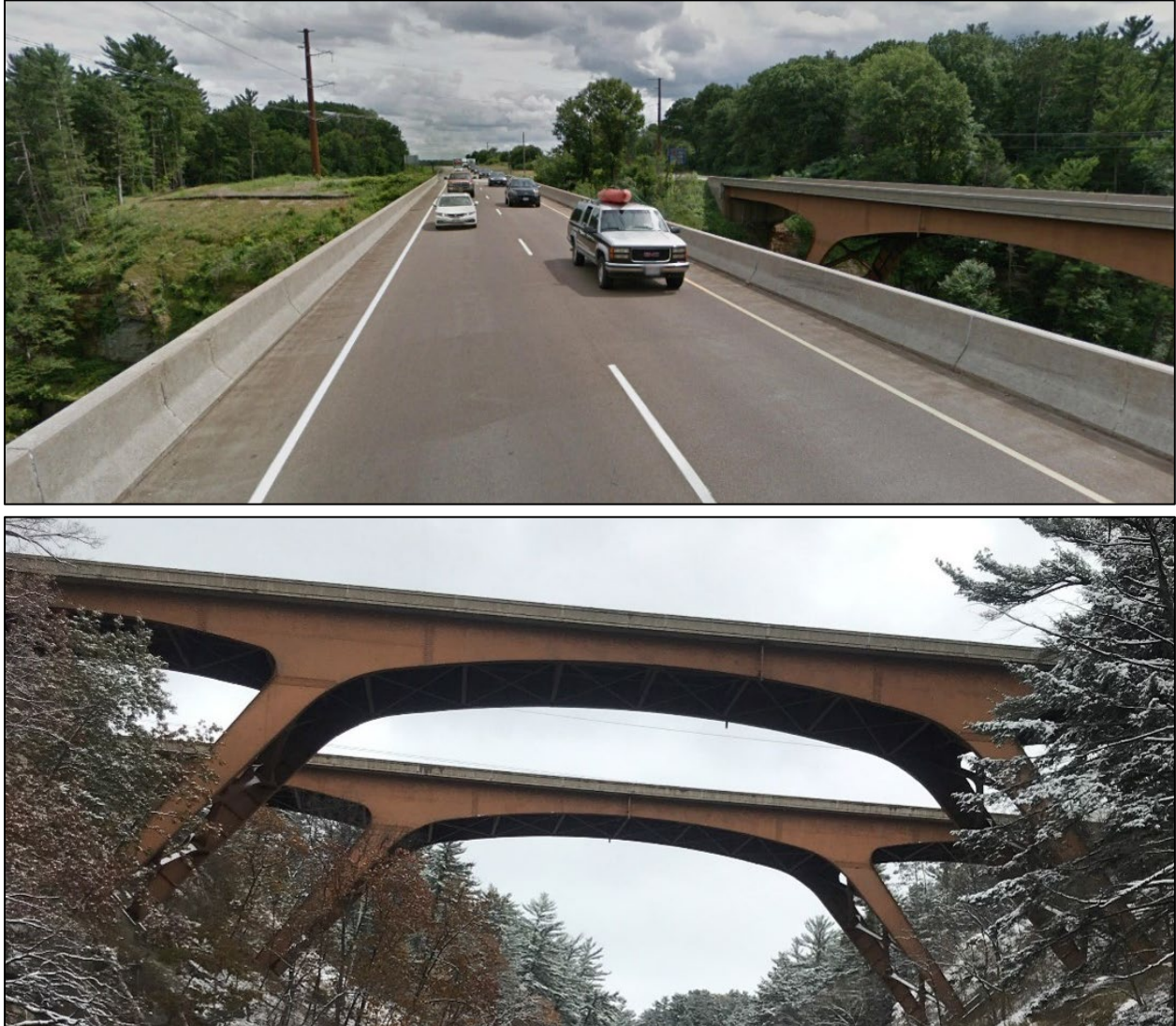
Figure 1-19: Mirror Lake Bridge Photos
