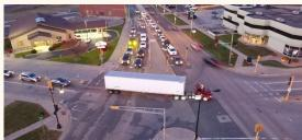
SIGNAL VISIBILITY: Most signalized intersections along US 53 & US 14/61 have no overhead indications or a single signal indication over the outside lane which can lead to signal visibility issues.
