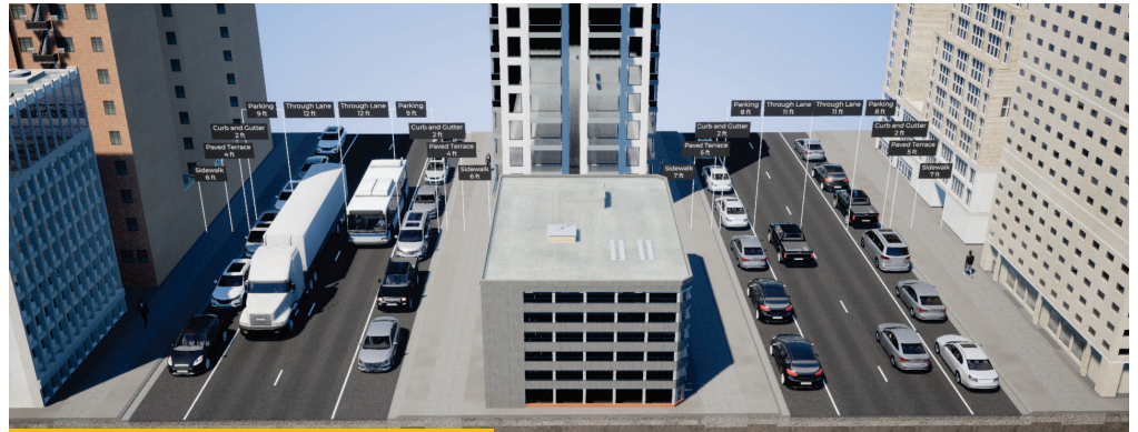
Existing Typical Section Total Width (Curb to Curb): 46 ft (SB US 53), 42 ft (NB US 53)
