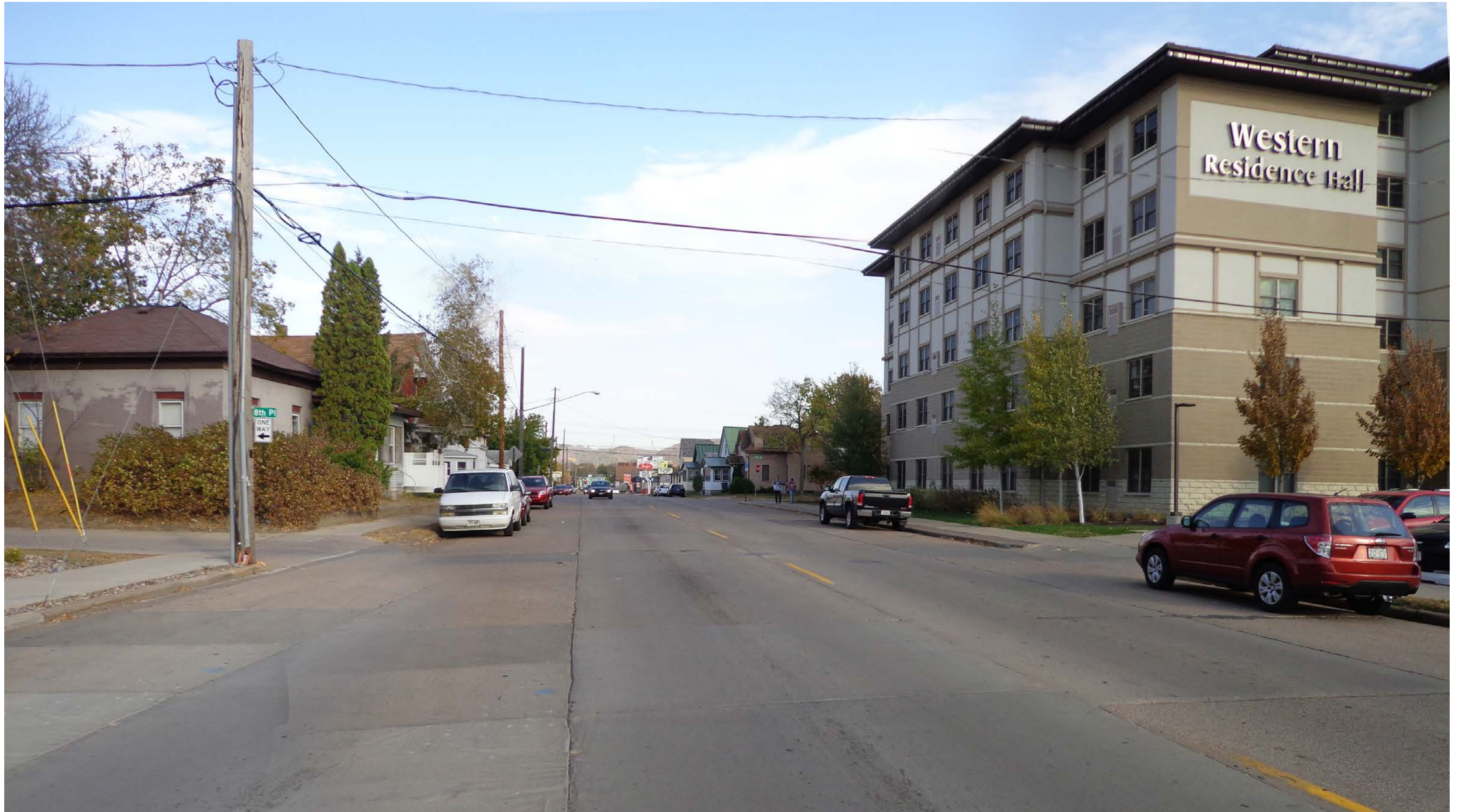
STRATEGY A1 (LA CROSSE STREET) EXISTING CONDITIONS
