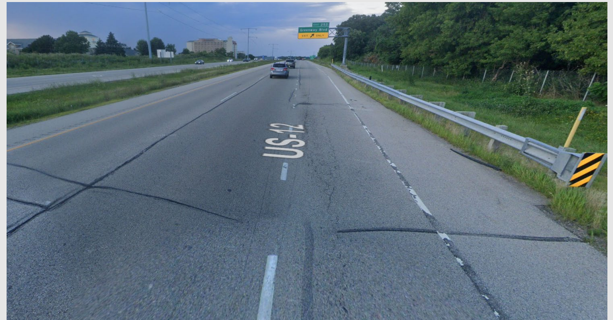
Deteriorating pavement; cracking and rutting, beam guard deficiencies, deteriorating guardrail, and substandard curb ramps
