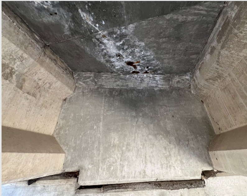
US 12/14 Westbound over Greenway Blvd (B-13-230) – spalling between girders and deteriorating bridge deck
