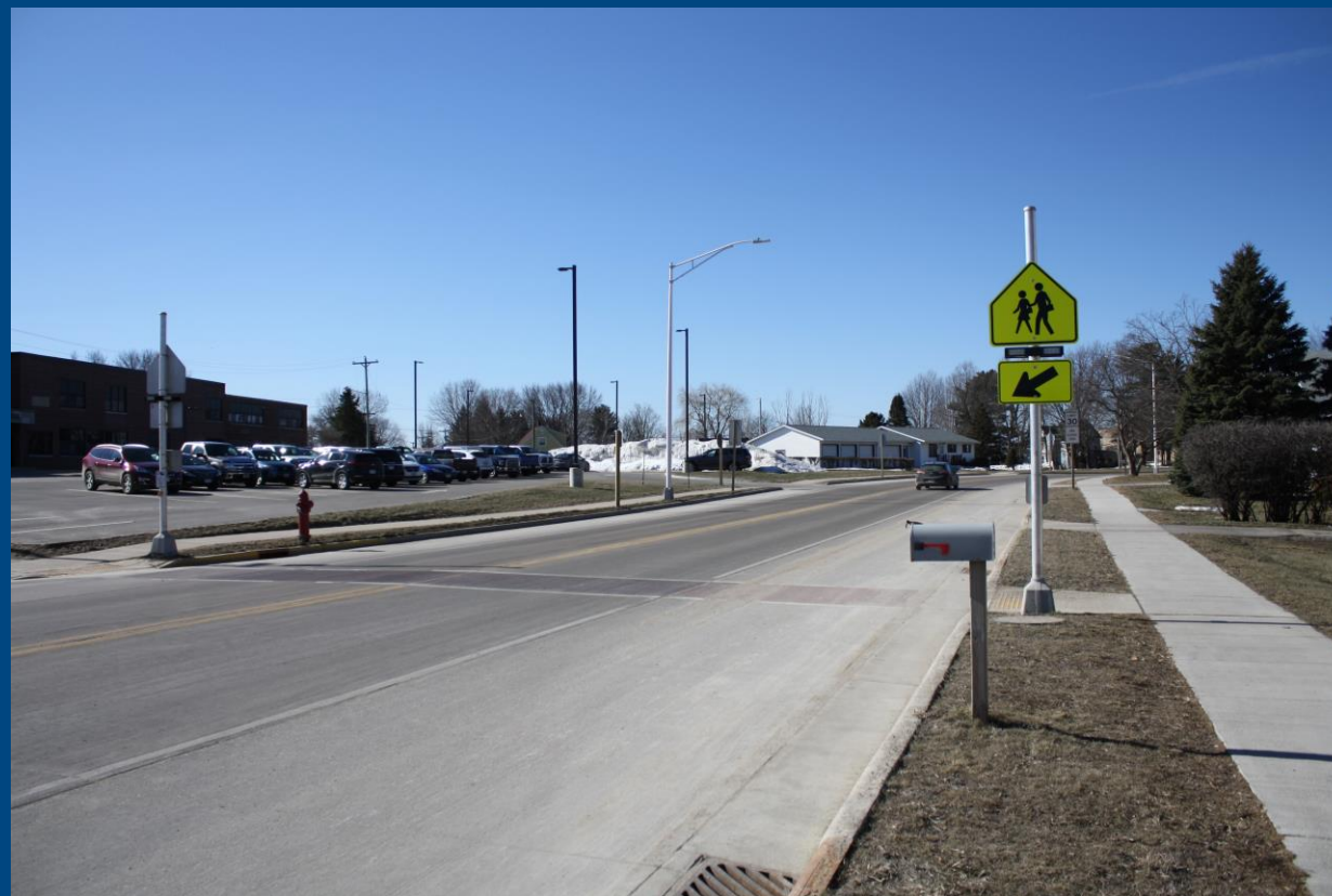
Example: Rectangular Rapid Flashing Beacon
