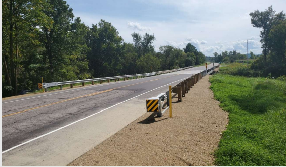
B-52-0067 Bridge over Bear Creek
