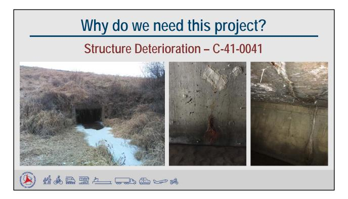
Another reason this project is needed is to rehabilitate structure C-41-0041. Structure C-41-0041 is a single-span reinforced concrete box culvert that is exhibiting spalling with exposed rebar and cracking with heavy efflorescence and rust staining throughout the structure.
