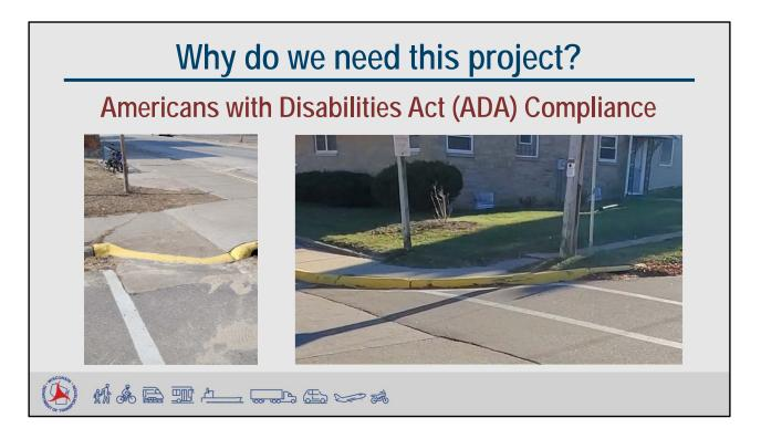
Another reason this project is needed is to replace non-ADA compliant curb ramps in the Village of Kendall. The current curb ramps along WIS 71 in the Village of Kendall either do not meet ADA slope requirements, are missing detectable warning fields, or do not have a curb opening at designated crosswalks.
