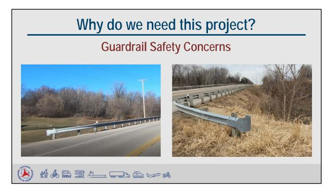
Another reason this project is needed is to replace the current outdated blunt end treatments and steel guardrail with Energy Absorbing Terminals (EAT) and MGS guardrail meeting current safety standards.
