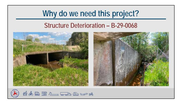
Another reason this project is needed is to rehabilitate structure B-29-0068. Structure B-29-0068 is a twin-cell reinforced concrete box culvert exhibiting cracking with rust staining, spalling along the waterline, and movement of the wings.
