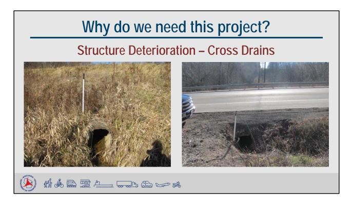
Another reason this project is needed is to replace deteriorated cross drains throughout the length of the project. The cross drains are corroded along the bottom and waterline, damaged around the ends, and distorted along the length of the pipes.
