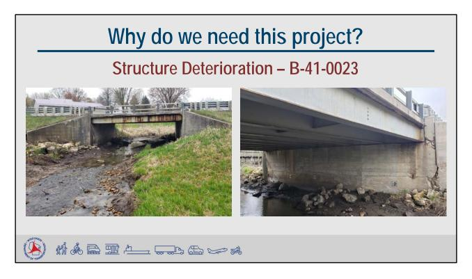
The final reason this project is needed is to replace structure B-41-0023. Structure B-41-0023 is a single-span steel girder structure that exhibits corrosion with section loss on the steel girders, spalling with exposed rebar, cracking and wearing on the concrete deck, spalling and cracking on the abutments, scraping and rusting on the metal railings, and movement of the wings.
