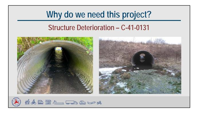
Another reason this project is needed is to replace structure C-41-0131. Structure C-41-0131 is a steel sectional plate pipe culvert that is exhibiting spalling of the concrete floor, settlement in the middle of the culvert, bulging throughout the length of the culvert, and scour around the ends of structure.
