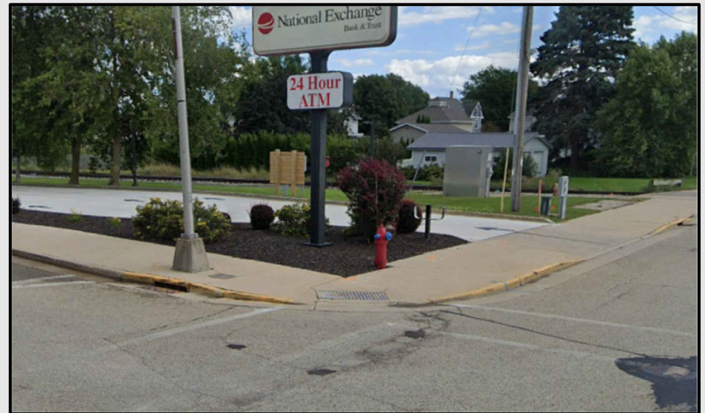
Example of non-compliant curb ramp on WIS 73
