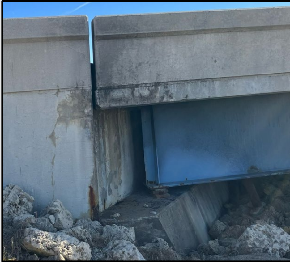
Existing condition of WIS 78 structure B-13-304 over US Highway 18/151
