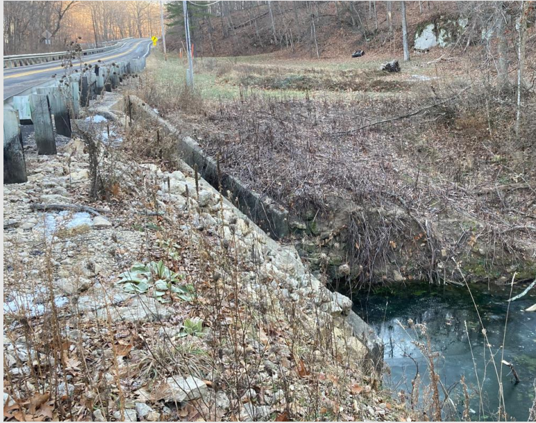
Box Culvert C-62-321–Outlet
