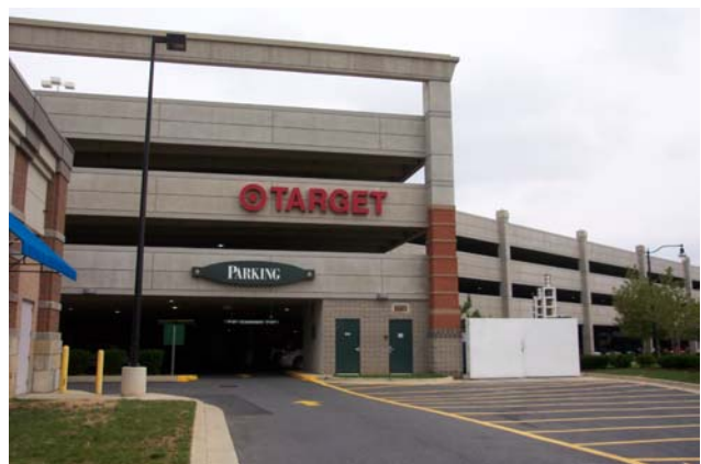
Washingtonian Center, a retail and entertainment center in Gaithersburg, Maryland, includes a large structured parking facility to accommodate the necessary parking. This view is of the back of the structure; the front of the structure incorporates retail uses on the first floors.
