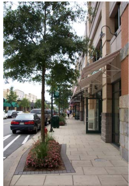
Washingtonian Center in Gaithersburg, Maryland, incorporates retail and commercial uses on the first floor of the parking structure.
