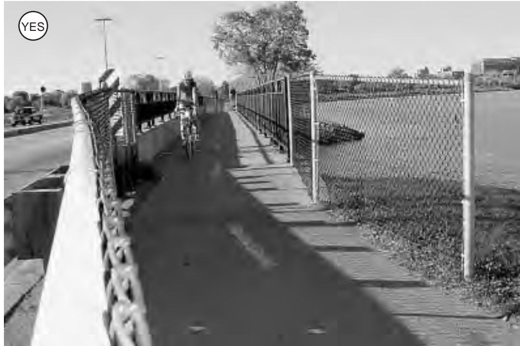
Figure 4-129: This retrofitted barrier-separated path bridge shares an existing roadway bridge's structure.
