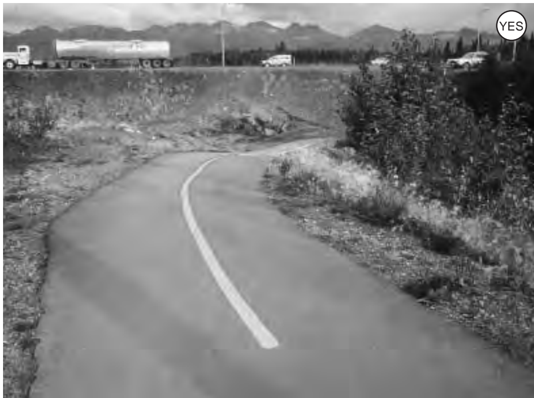
Figure: 4-26: An example of centerline striping used in a curve to separate bicyclists going opposite directions. In this case, no curve widening was used, however vegetation has been trimmed back to improve sight lines.
