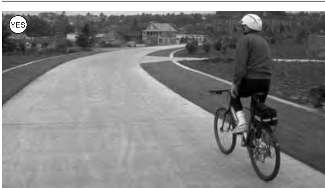
Figure 4-44: Concrete can provide a smooth and long-lived surface, as shown on this shared-use path.
