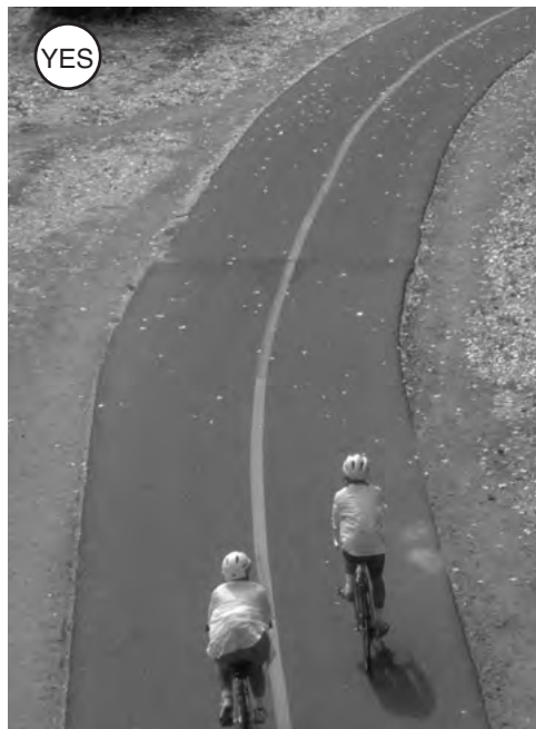
Figure 4-1 (left and right): Shared-use paths often serve as necessary and important extensions to the roadway network.
