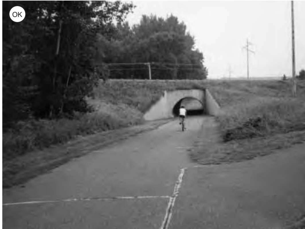
Figure 4-88: A grade separation takes bicyclists under a moderately busy highway. Sightlines are good and the entry and exit grades are slight.
