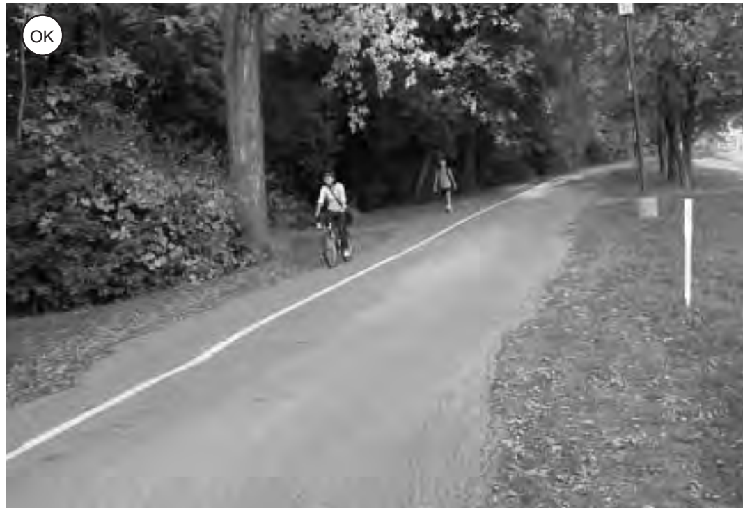
Figure 4-60 (right): One approach to separating bicyclists and pedestrians. Expect only modest success with treatments that do not physically separate bicyclists and pedestrians.
