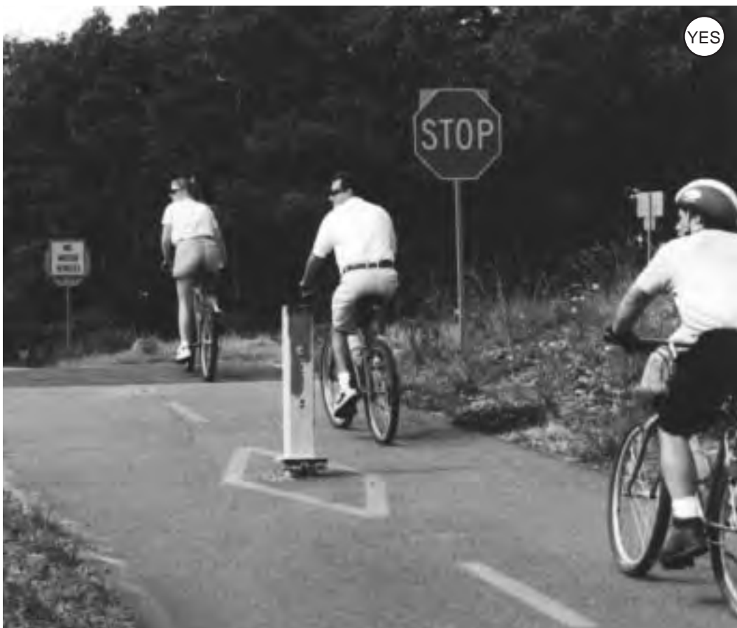
Figure 4-98: An at-grade path crossing of a low-volume rural roadway. Note damage to bollard; see Section 4.17.3 for alternative approaches to discouraging motor vehicle intrusion.
