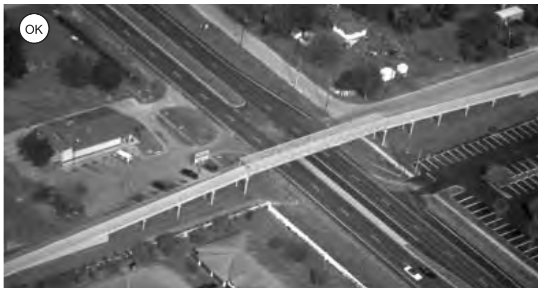
Figure 4-114: Overpass approach ramps are typically longer than ramps for underpasses and can significantly increase costs.
