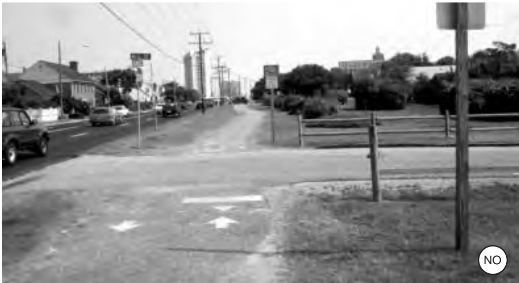
Figure 4-110: Positive features of this crossing are good visibility and proximity to the roadway intersection. Problems include lack of crosswalk marking and confusing right-of-way assignment (bicyclists apparently required to yield to motorists who have a stop sign).
