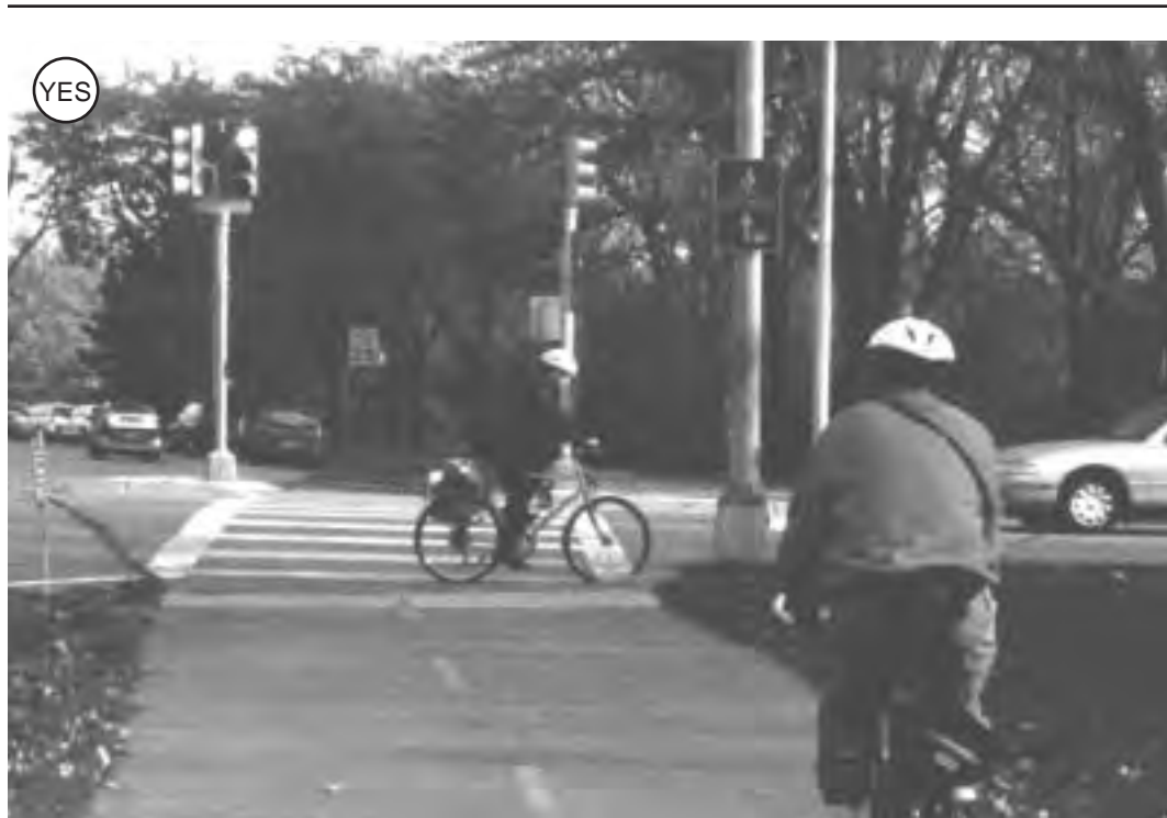
Figure 4-106: An urban crossing that takes advantage of an adjacent signalized intersection. A bicycle signal loop detects bikes to change the signal. Note high-visibility crosswalk marking.
