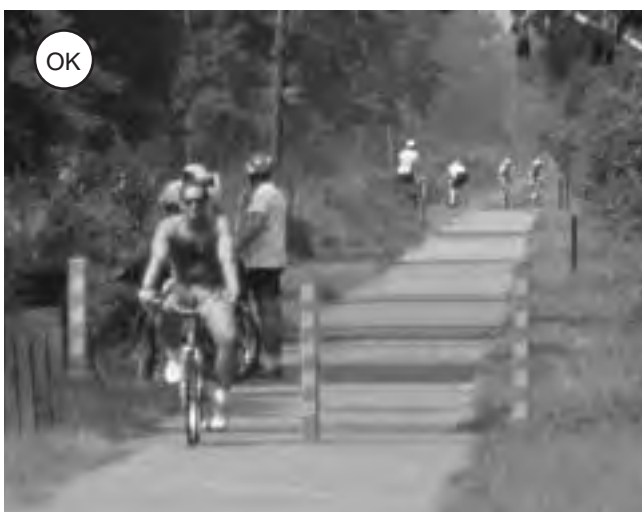
Figure 4-151: If bollards are necessary, they should be reflectorized, positioned in a highly visible location, and separated by 5 ft. (1.5 m).
