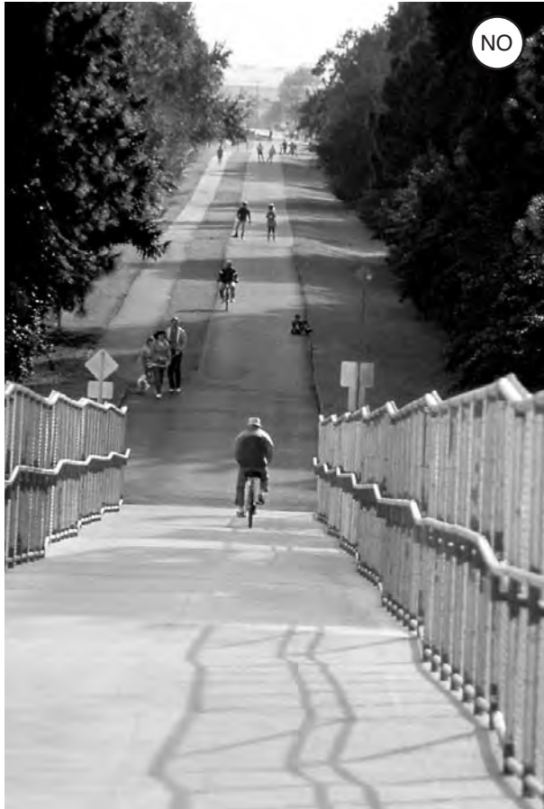
Figure 4-122: While this ramp provides landings and meets ADA slope limits, the overall length and height make it impossible to use for many disabled people.
