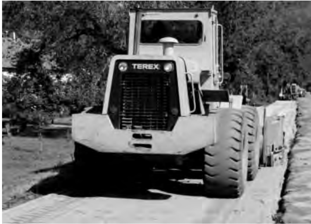
Figure 4-41: Preparing shared- use path subgrade.
