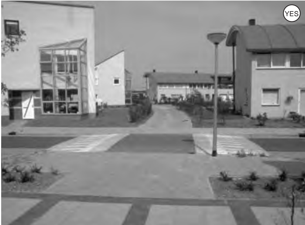
Figure 4-97: A raised path crossing used to slow motorists and give path users priority.
