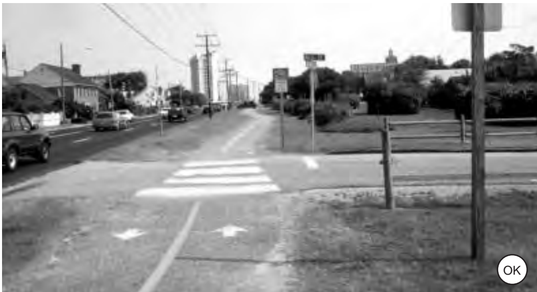
Figure 4-111: Some elements that would help include highlighting the crossing, moving the stop sign and stop bar for the crossroad, as well as adding appropriate warning signs (not shown). Still, motorists will tend to stop in the crosswalk to wait for traffic and the design is far from optimal.
