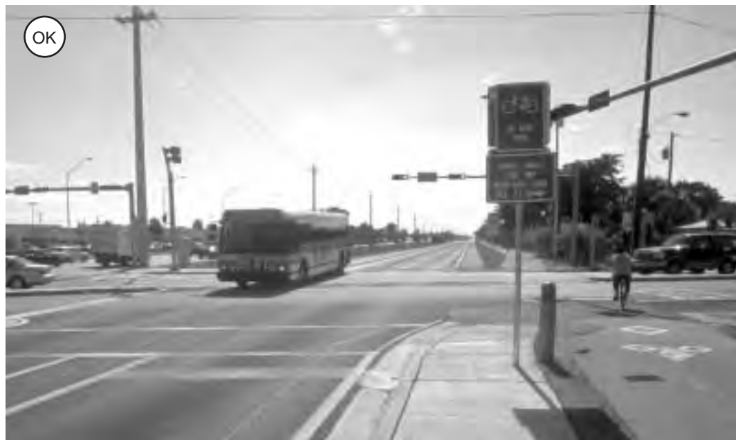
Figure 4-109: This path has few crossings and good visibility at this intersection. Even so, it is important to reduce conflicts between turning and crossing movements. A separate left turn phase for the bus, for example, could help.
