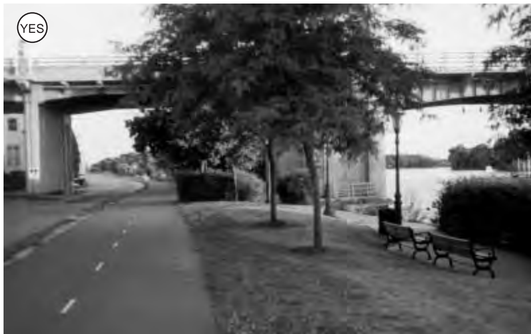
Figure 4-113: Near riverfronts, it is often possible for a “natural” grade separation to occur where roadways pass overhead. Adequate clearance must still be allowed for path users and maintenance vehicles.
