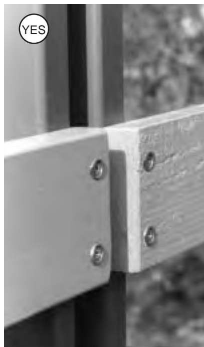
Figure 4-121: A simple rub rail mounted at handlebar height can divert out-of-control bicyclists back onto the pathway.
