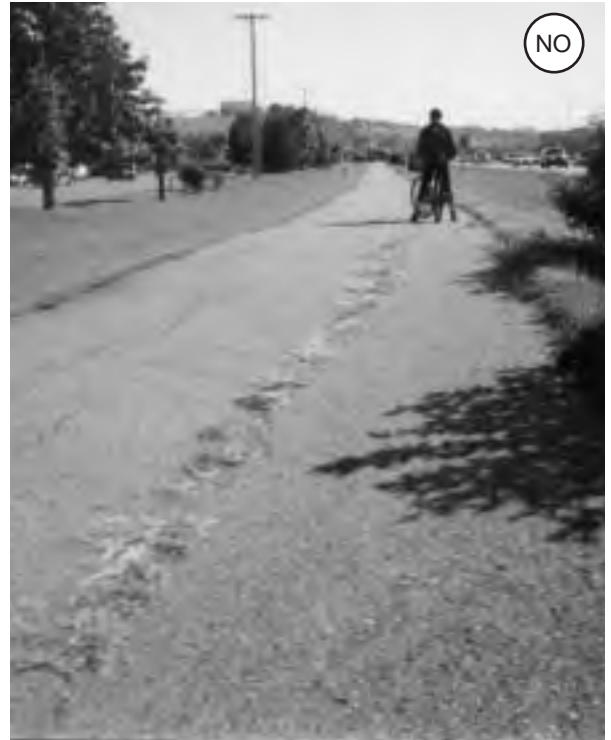
Fig. 4-39: Weeds break through a relatively new path.
