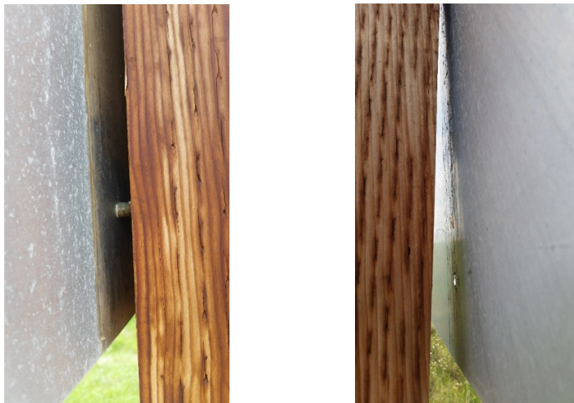
Figure 1: Back side of an aluminum sign after 2 years
