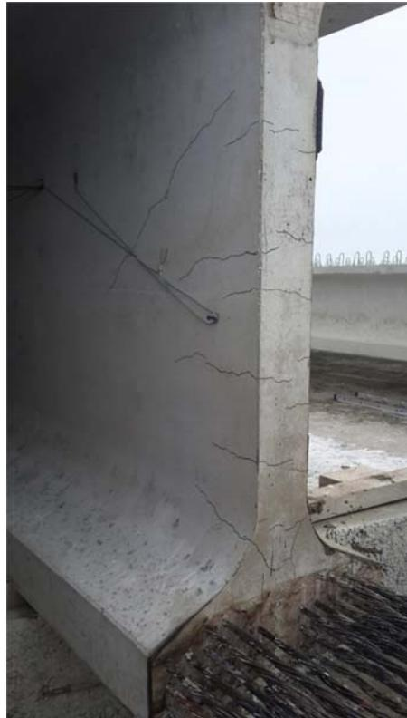
Figure 1-1. Cracks at the end of a Wisconsin 72W girder.
