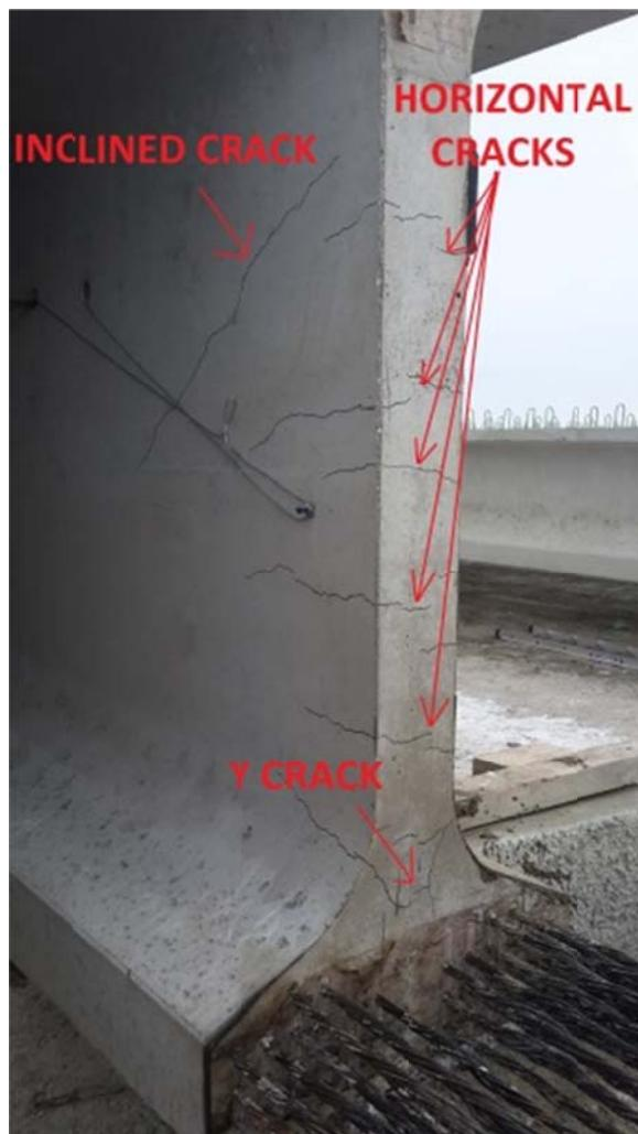
Figure 3-3. Inclined, Horizontal Web, and Y cracks shown on 72W girder.
