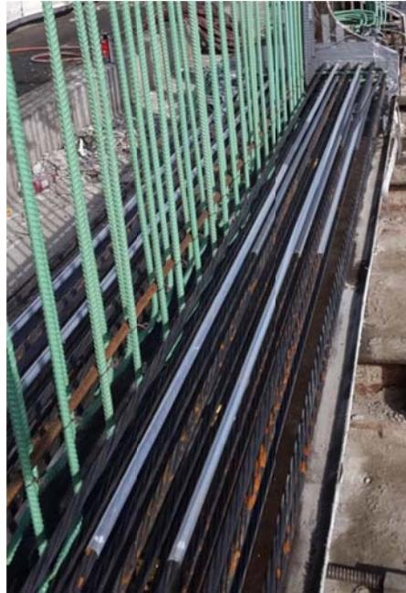
Figure 5-5. Plastic shield around strand for de-bonding.
