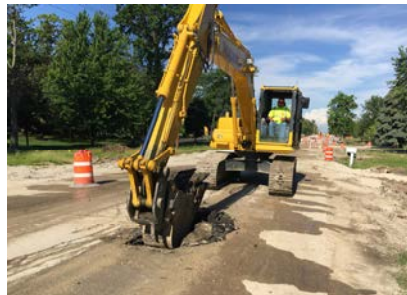
(e) Pavement surface removal at Edgerton Ave
