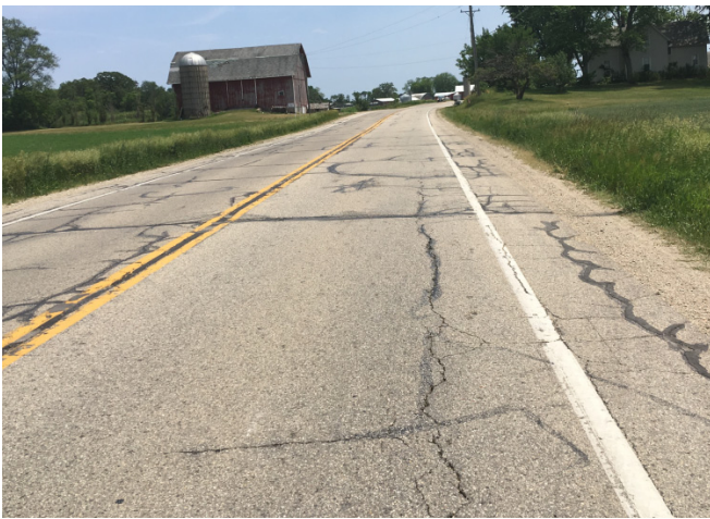
c) Pavement surface distresses
