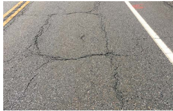
(f) Fatigue and block cracking
