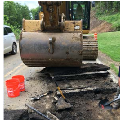
(c) Pavement surface removal at STH 162
