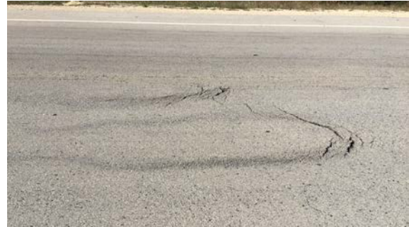
(b) Delamination (slippage)
