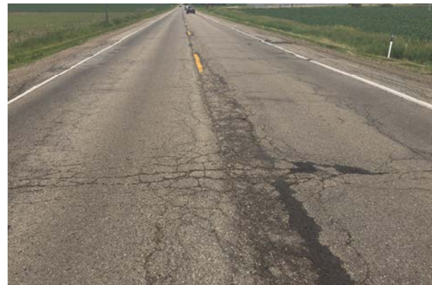
(h) Fatigue cracking
