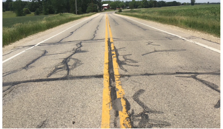
b) Pavement surface distresses
