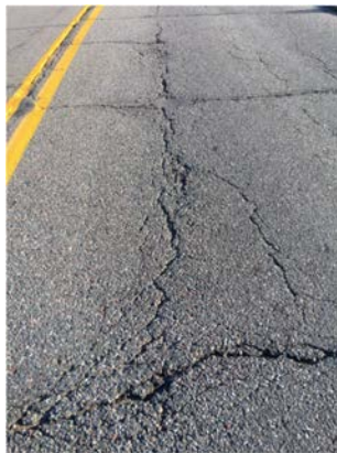
(g) Fatigue cracking
