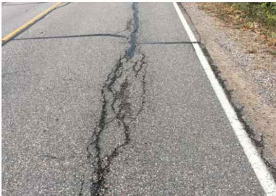
(e) Fatigue cracking and transverse cracking
