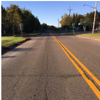
c) Pavement surface distresses
