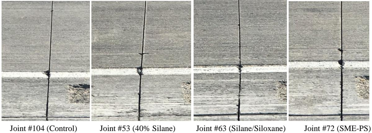
**Figure 5.4 Examples of small spalling observed during the August site visit**
