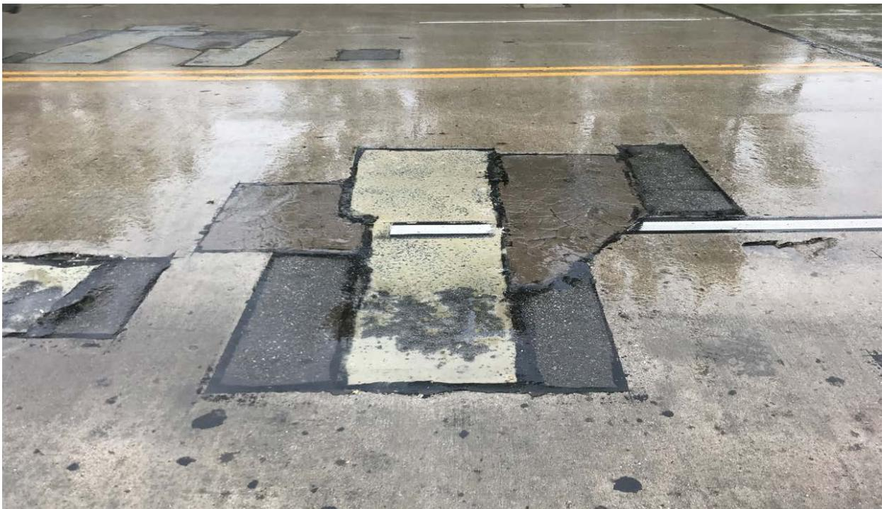
Figure E-25. RM-4 PDRs on bridge deck with starkly different colors
