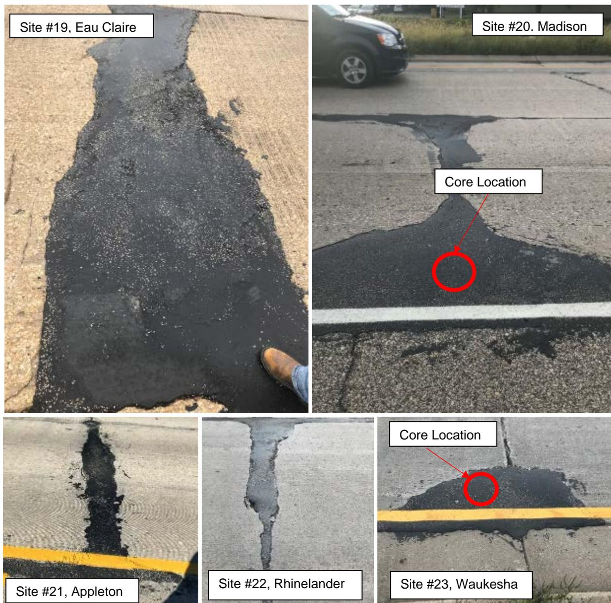
Figure 3-22. RM-5 used in concrete pavement PDR applications.
