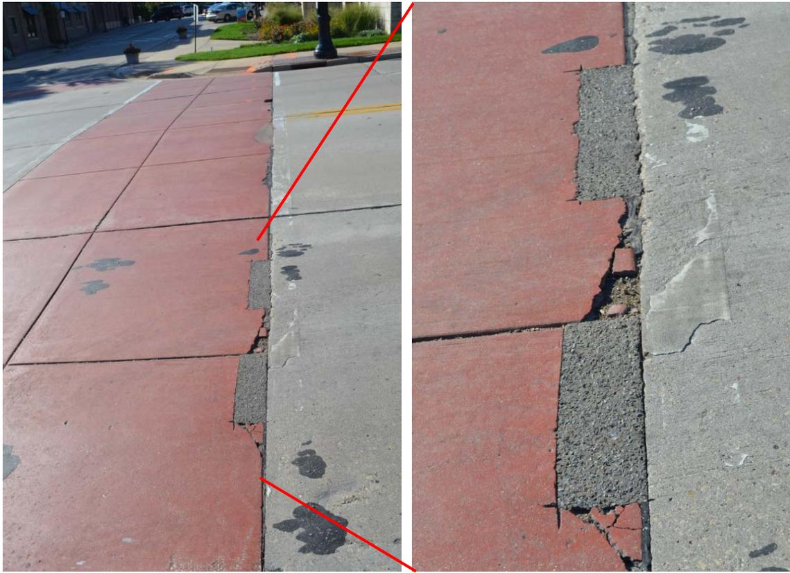
Figure E-1. PDRs along transverse joint
