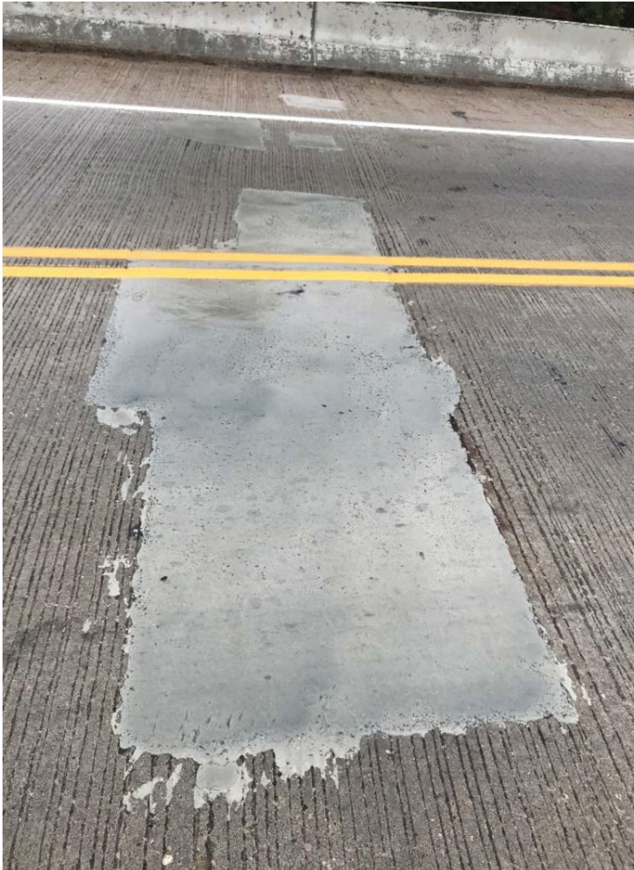
Figure E-20. PDRs on bridge deck (2)
