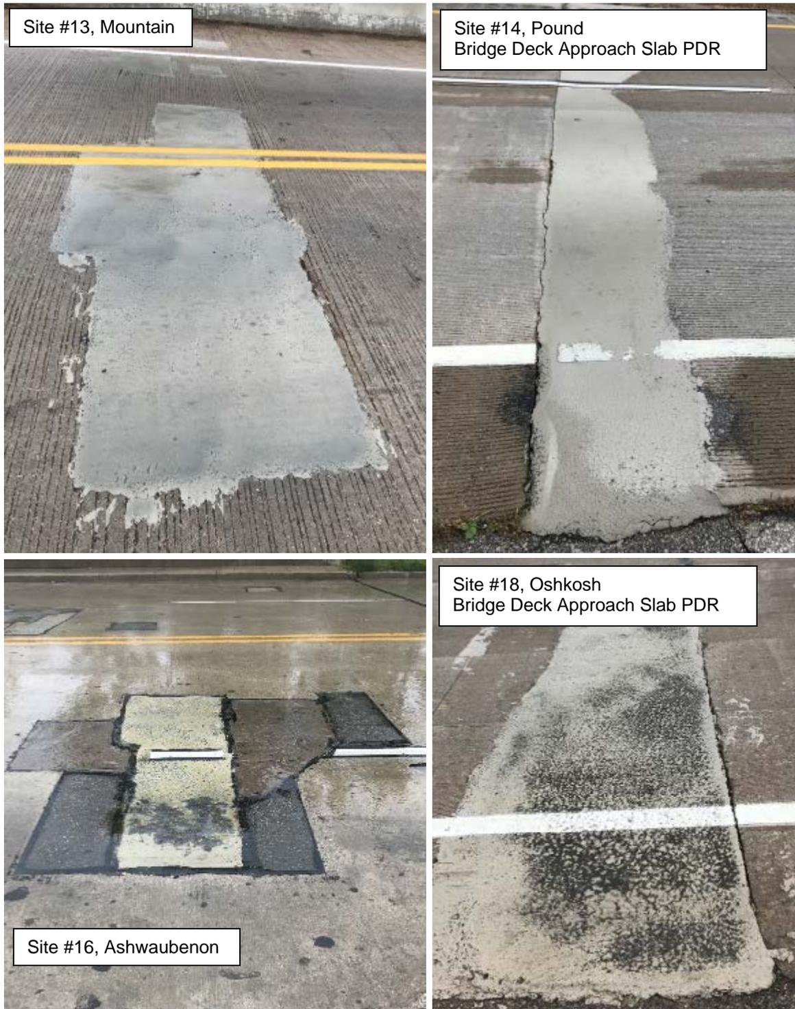
Figure 3-19. RM-4 used in bridge applications.
