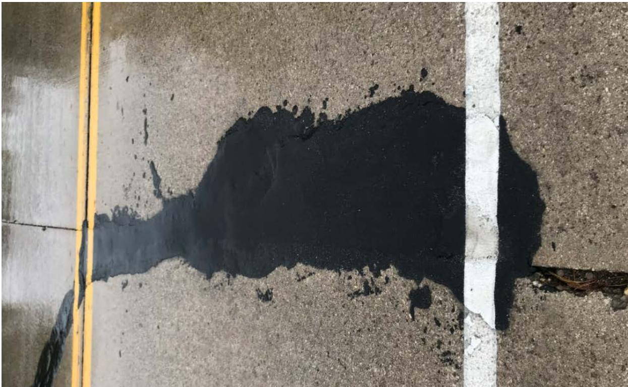
Figure D-6. PDRs along transverse joint
