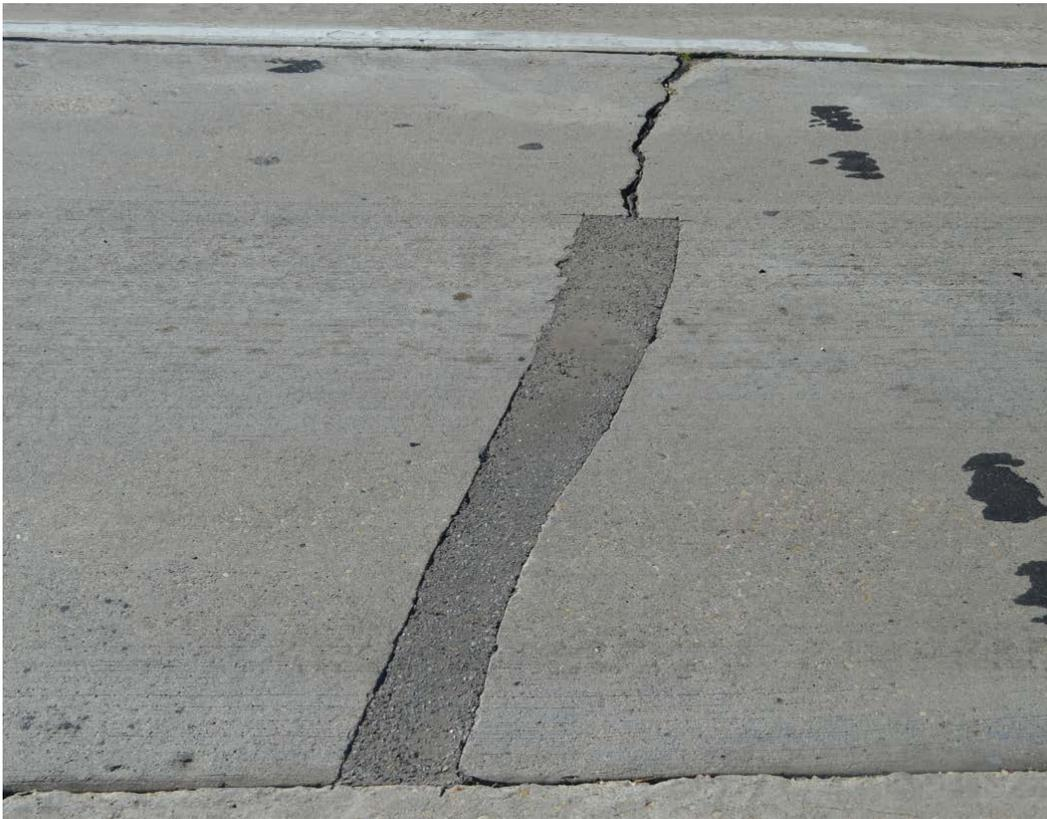
Figure E-3. PDR over a transverse crack
