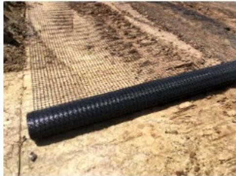
Geogrid material and aperture shapes vary by manufacturer, and there are multiple test methods for determining strength. WisDOT currently uses ASTM D4595, which was originally developed for geotextiles, a different type of geosynthetic. ASTM D6637 Method B has gained popularity, as agencies and
