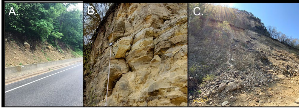
Representative photos for each of the three hazard mechanisms identified along the study corridor (A. Rockfall B. Fragmental rockfall and rockslides C. Shallow colluvial slides). Photos from BCG Engineering.
