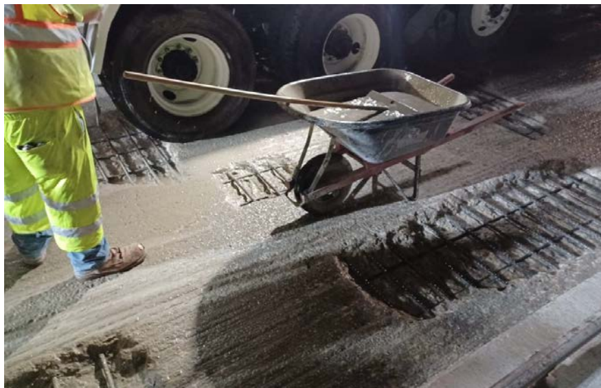
Figure 18. Application of cement-water slurry before overlay placement.
