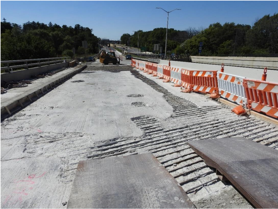
Figure 16. Bridge B40-336 before placement of new overlay.
