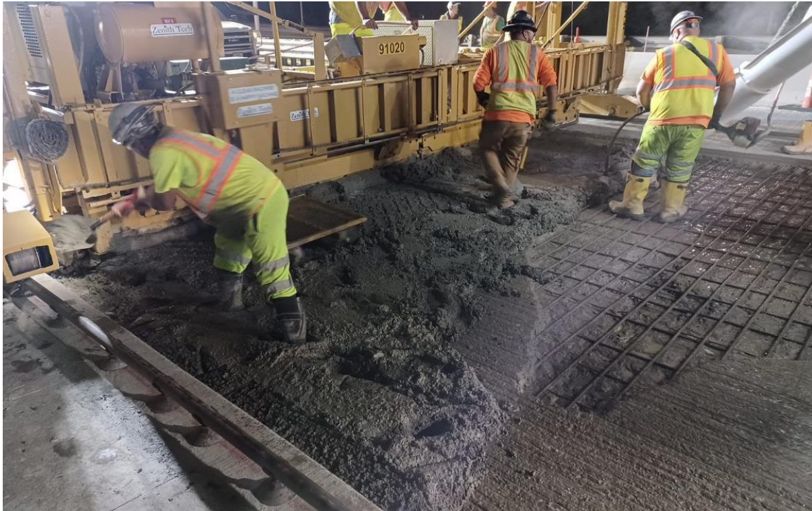
Figure 19. Placement of overlay using double vibrating screed.
