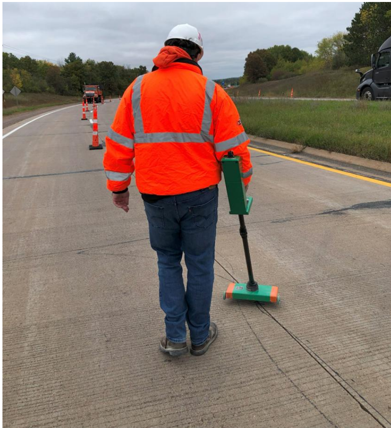
Figure 5. MIT-SCAN-T2 testing to locate tie bar in Chippewa County STH 178 NB.
