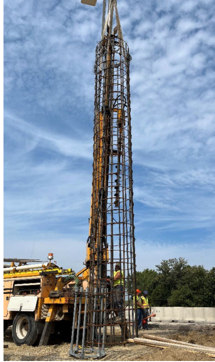
Figure 3-10 : Placing reinforcement cage for S-13-570
