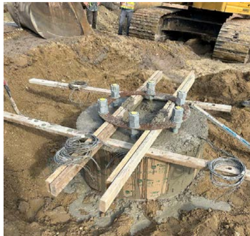
Figure 3-11: Fixing anchor bars in S-13-570
