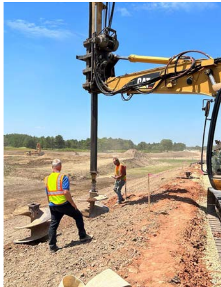
Figure 3-9. Excavation of the hole using excavator-mounted drilling machines
