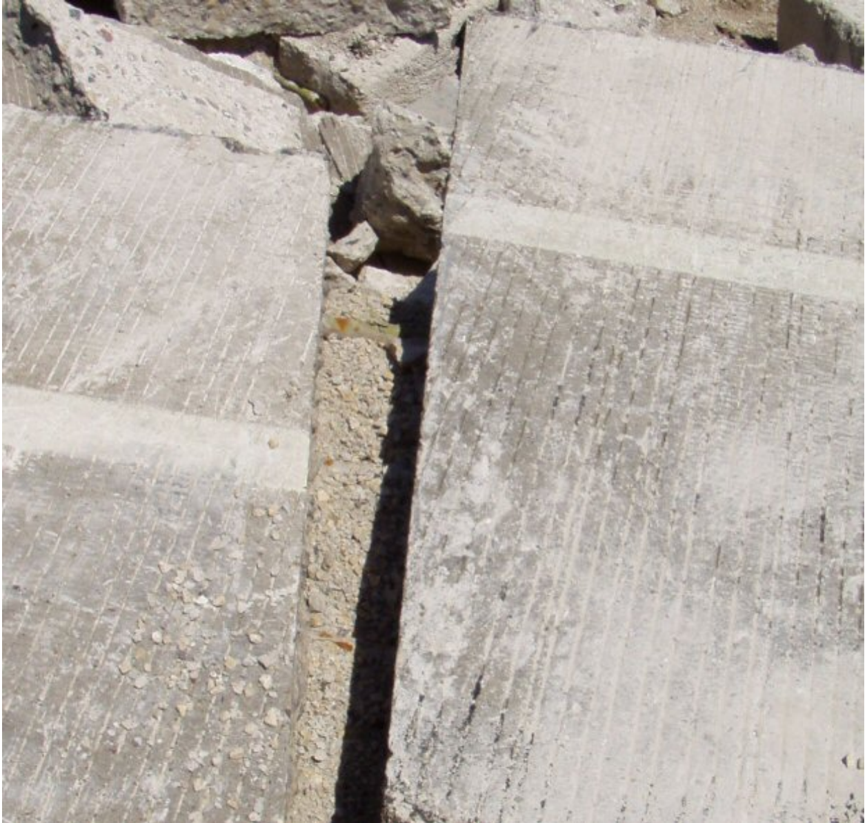
Figure 8. Slab corner without surface distress, but showing delamination of acute corner at mid depth.
