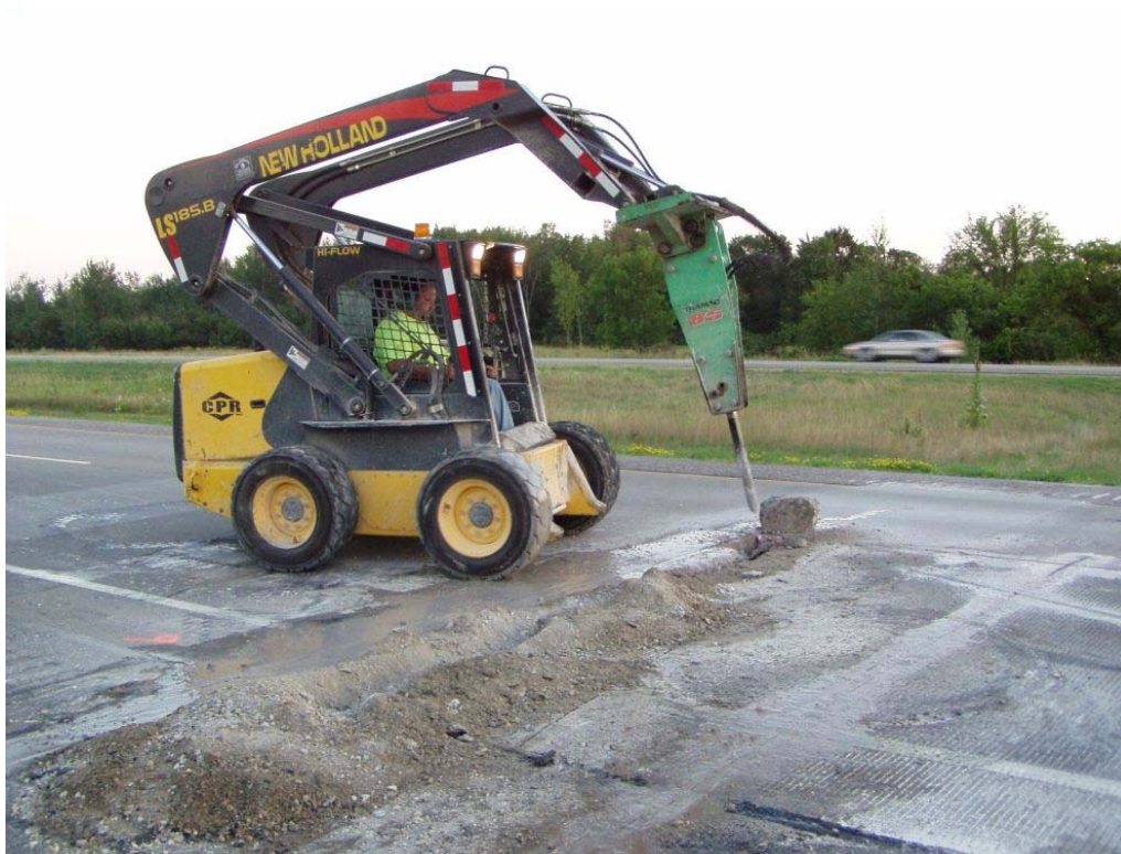
Figure 2. Removing corner of repair area.
