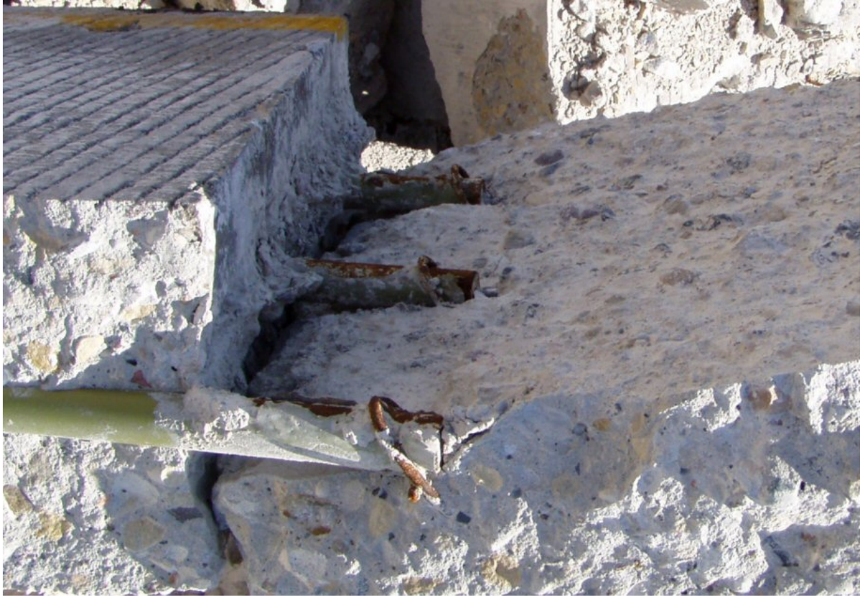
Figure 9. Distressed slab corner showing delamination of acute corner at mid depth. Note differences in dowel condition on acute corner (right) versus obtuse corner (left).
