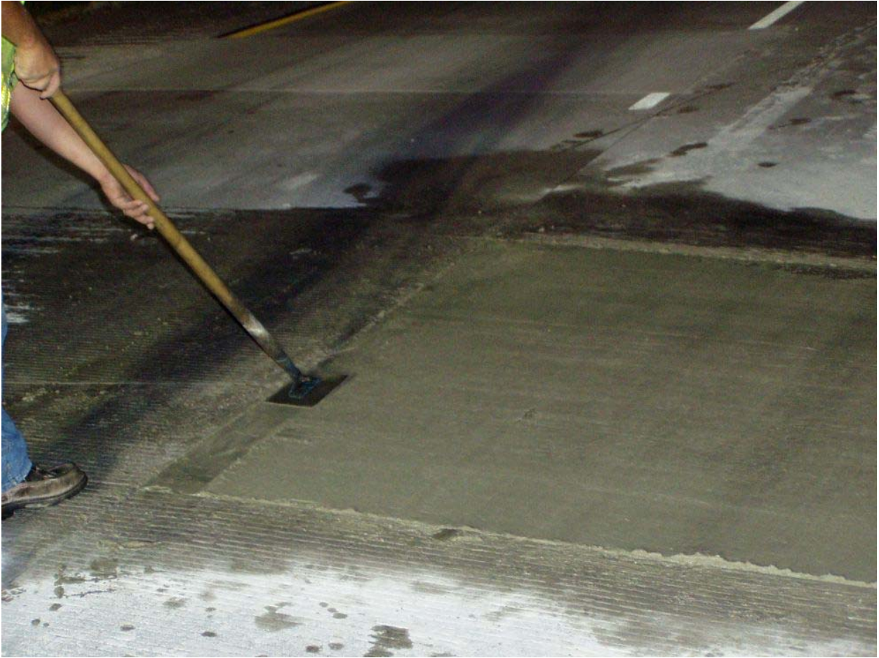
Figure 6. Patching repair area using fast-track concrete.
