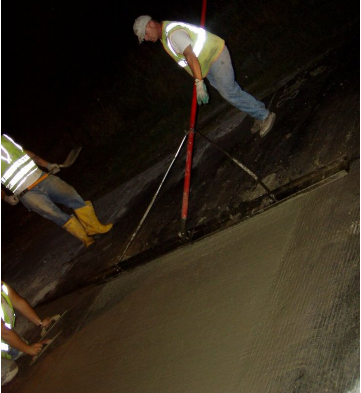
Figure 5. Patching repair area using fast-track concrete.
