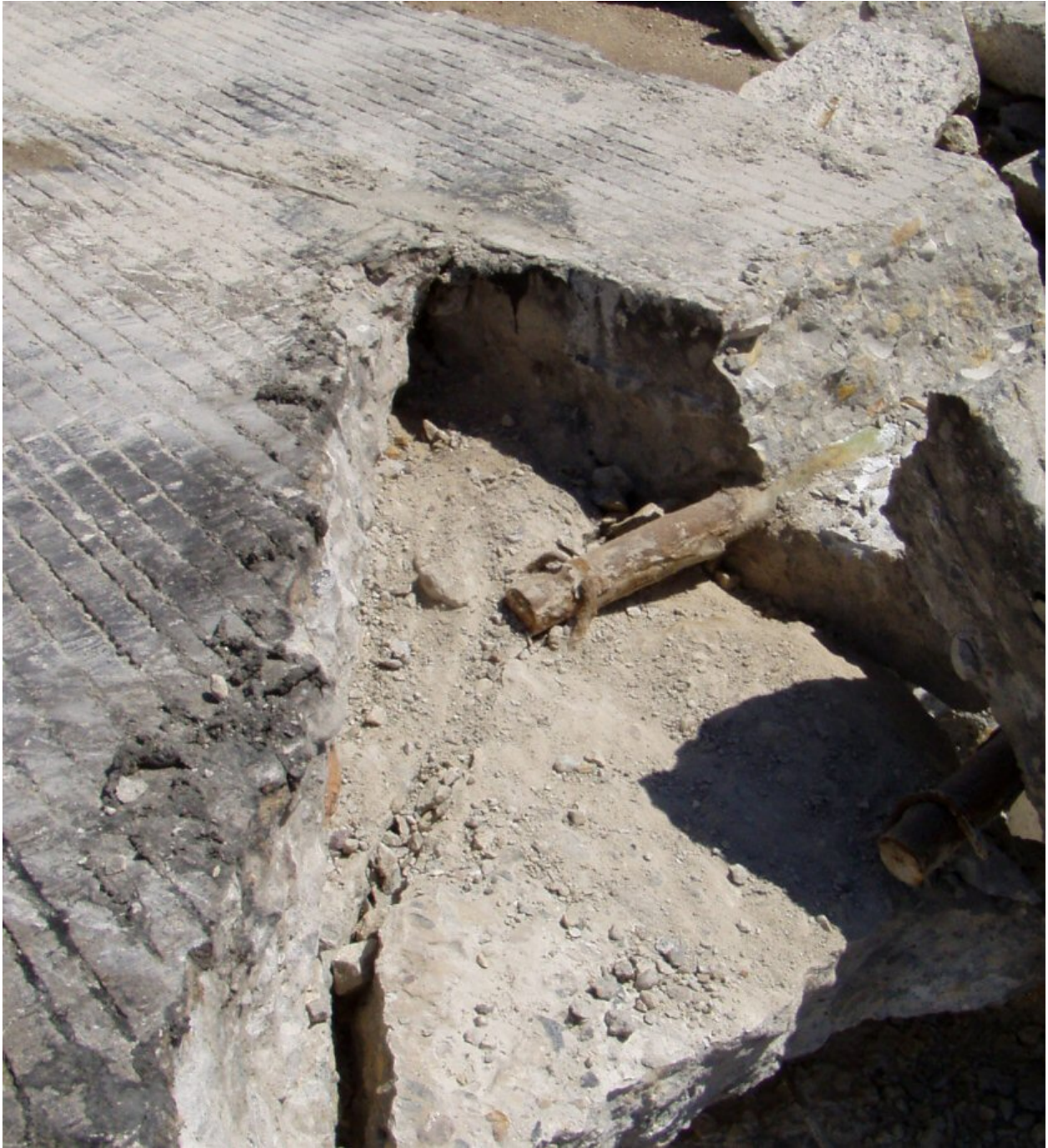
Figure 7. Distressed slab corner showing delamination of acute corner at mid depth.
