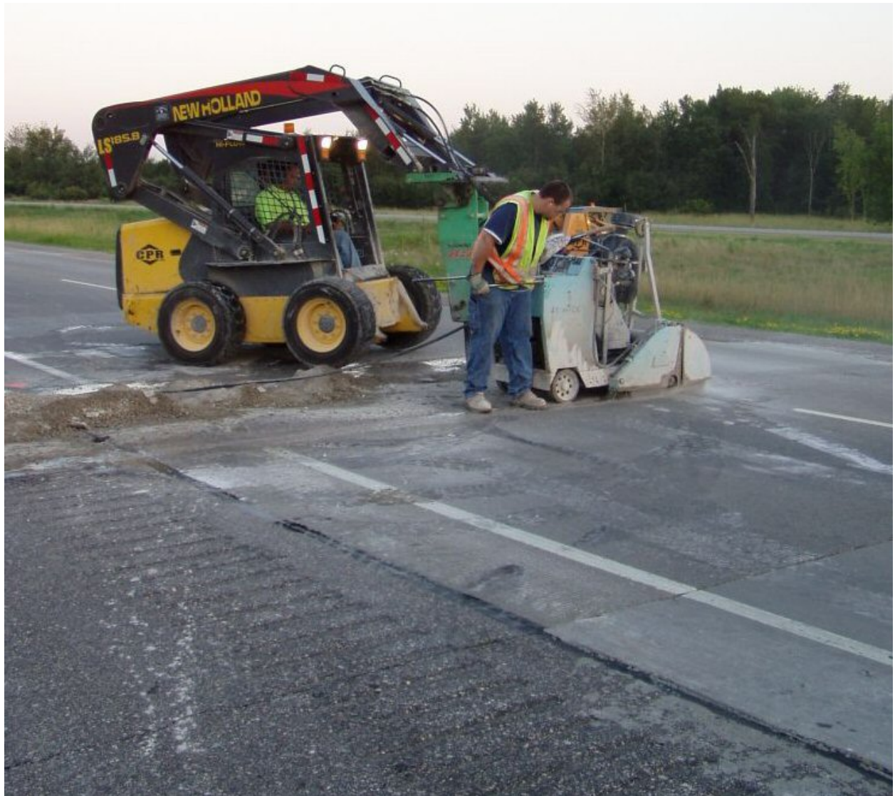
Figure 1. Sawing on both sides of repair area (flanking distressed joint).
