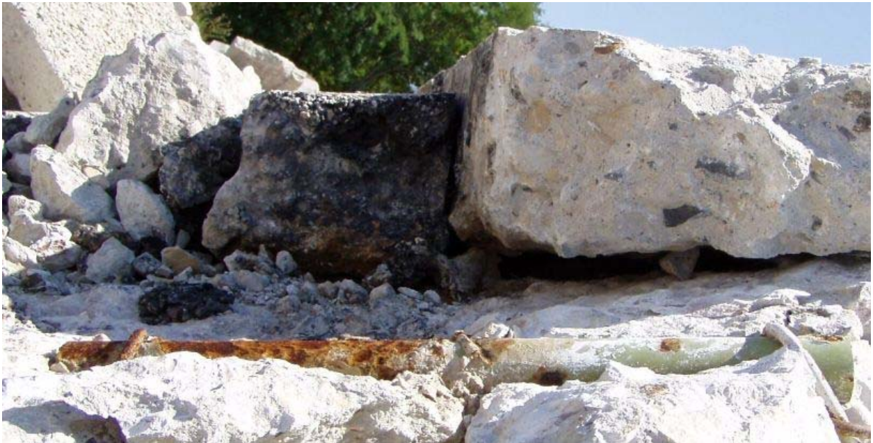
Figure 10. Side view showing dowel bridging distressed corner. Note differences in dowel condition on acute corner (left) versus obtuse corner (right). Note crack repair material infiltration.
