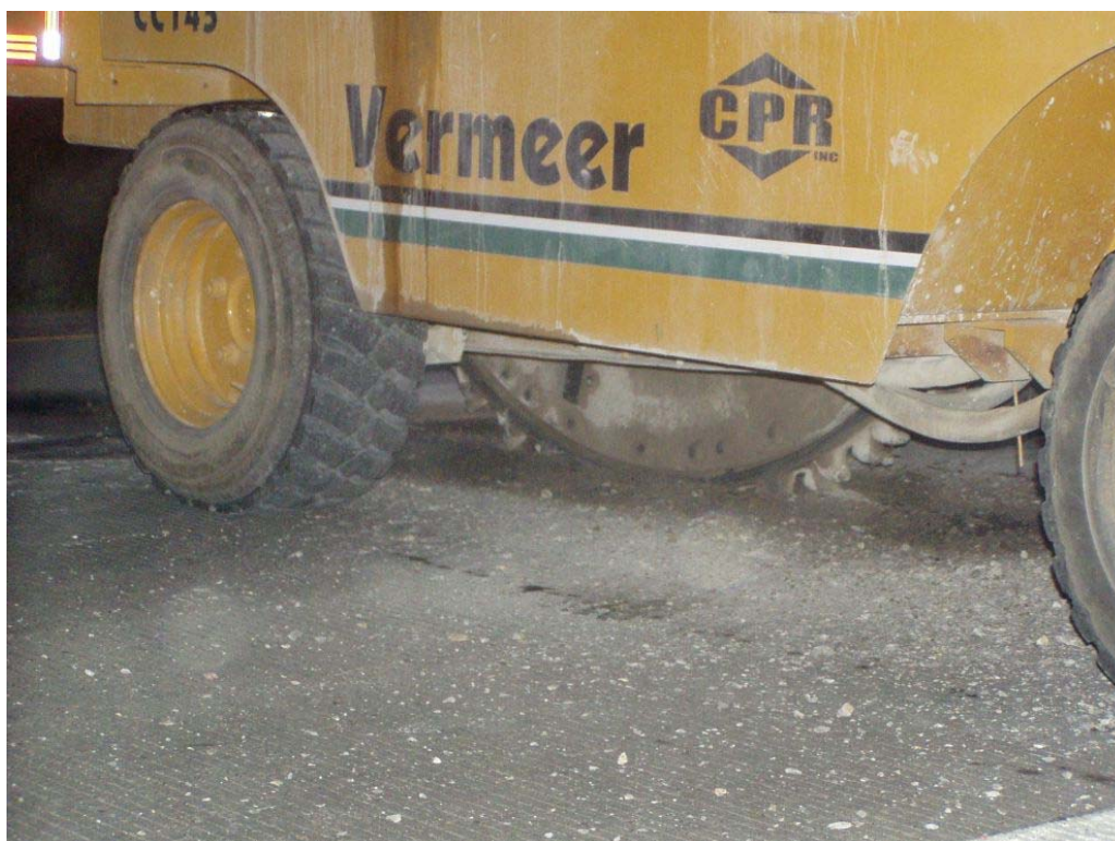
Figure 3. Concrete cutter to remove edge of repair area.
