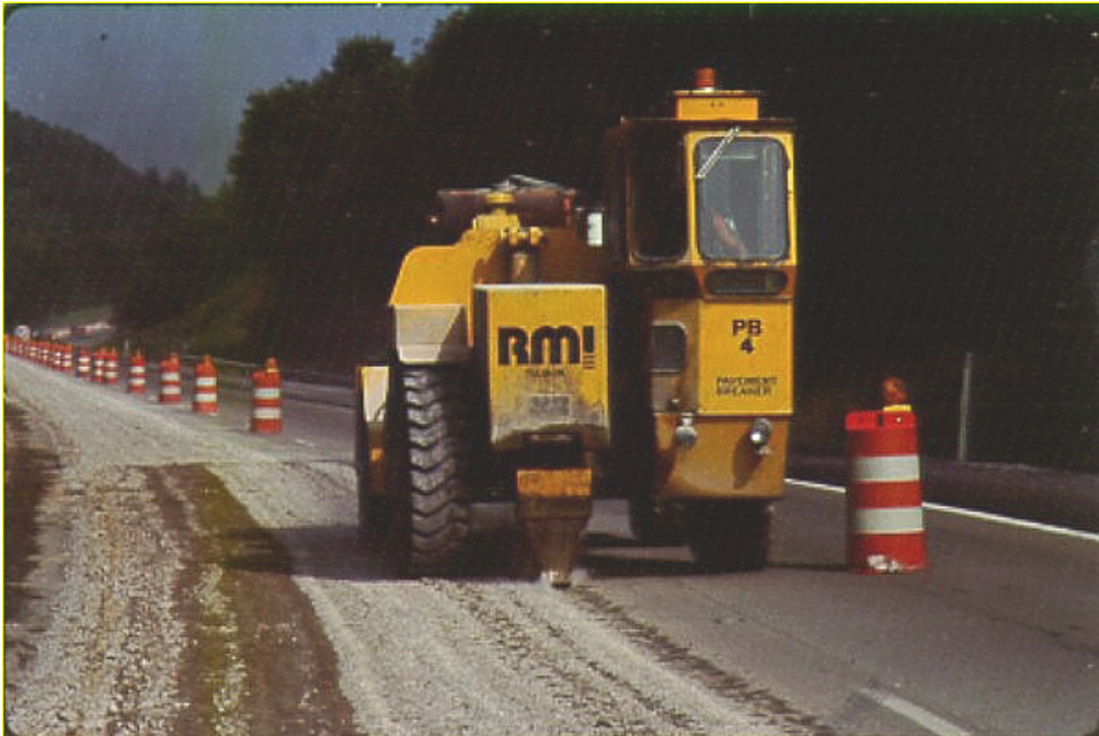
Figure 7 Photo of the resonant frequency pavement breaker for rubblizing PCC slabs.
