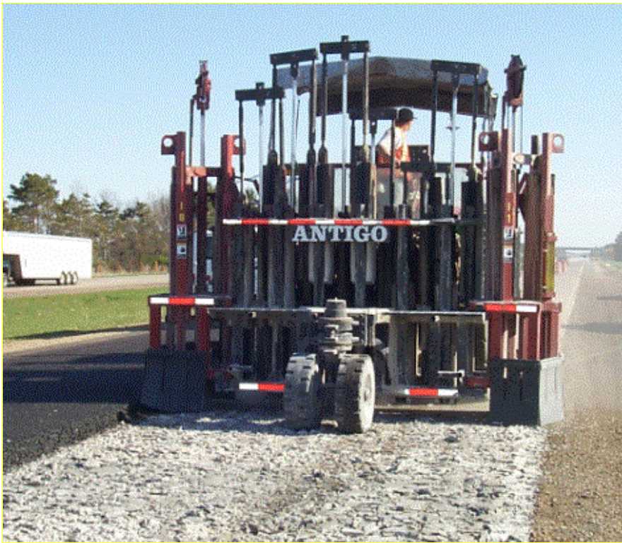
Figure 8 Photo of the multiple drop hammer for rubblizing PCC slabs.
