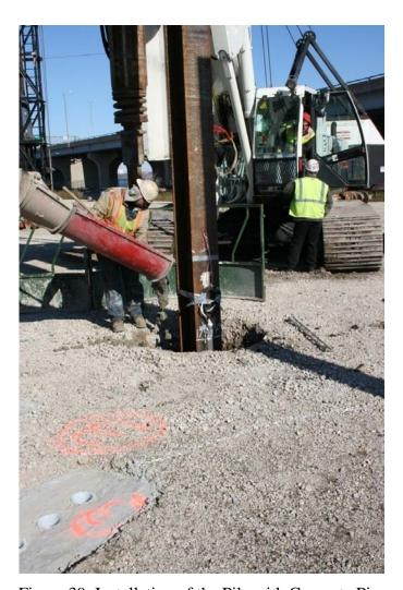
Figure 39: Installation of the Pile with Concrete Pier
