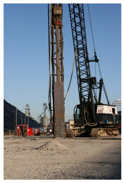
Figure 28: Installation of the Pile with Steel Plate
