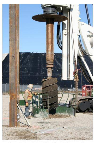
Figure 37: Installation of the Pile with Concrete Pier
