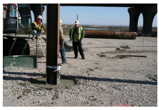
Figure 40: Installation of the Pile with Concrete Pier
