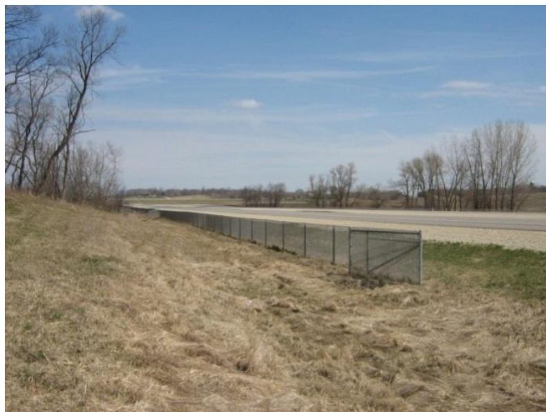
Figure 35 Turn-Around Turtle Fencing Photo Credit: Stacy Cook
