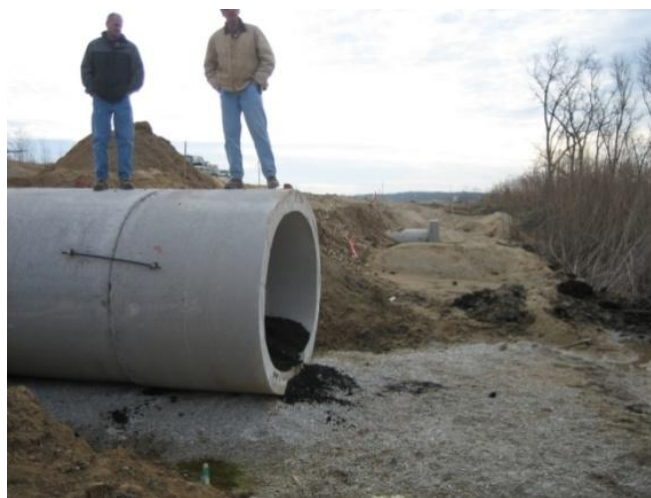
Figure 5 Installation of Ecopassage Photo Credit: Gary Birch, WisDOT
