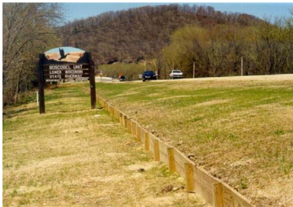
Figure 17 New Turtle Barrier Photo Credit: Bob Swartz
