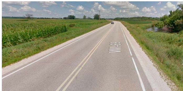
WIS 69 prior to reconstruction
