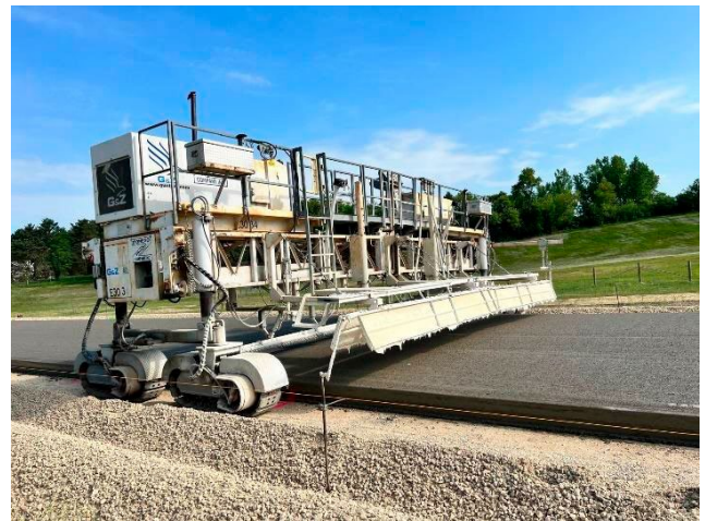
Field test construction on WIS 15
