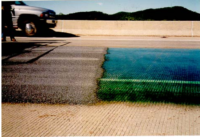
Photo 2: Italgrip® resin before and after aggregate application
