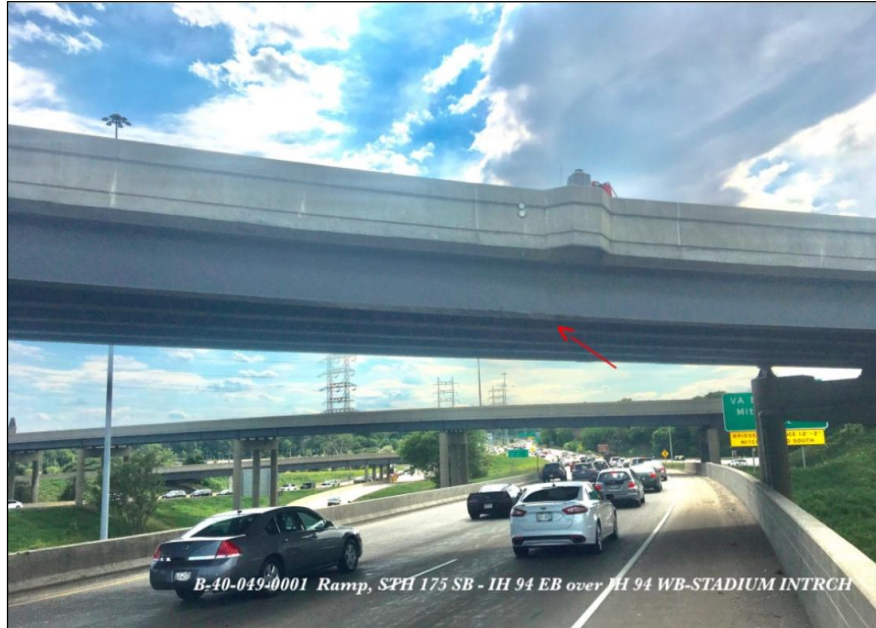
Figure 1.1.1.6-2: Photo showing location of damage in context of roadway. From this, right lane and shoulder closure would be required to repair the area with the arrow. Additional closer photos also would be required. Ideally this would be taken at an angle that clearly shows position relative to lane, but traffic did not allow.
