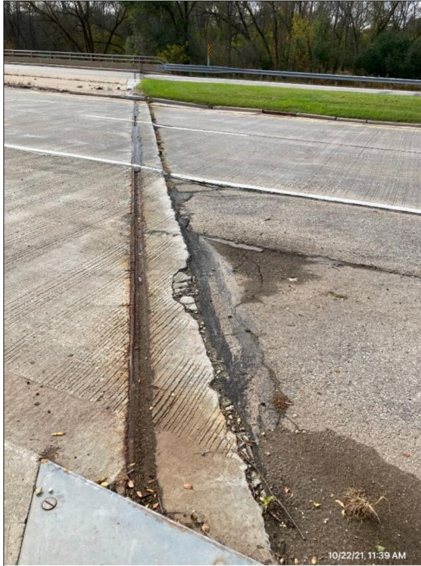
Figure 1.1.1.6-1: Good maintenance photo showing damage, location, and extent of header damage in shoulder. Provide notes to support photo. For repair of asphalt paving, additional photos of extents would be useful.
