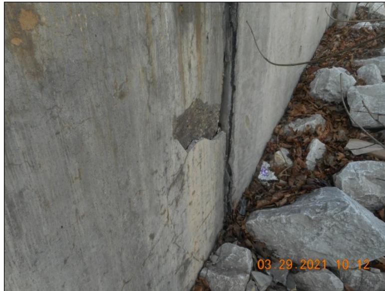
Figure 1.1.1.5-3: Good scale on photo: Leaves, riprap, trash present for scale, taken at angle that shows size of spall and offset of joint
