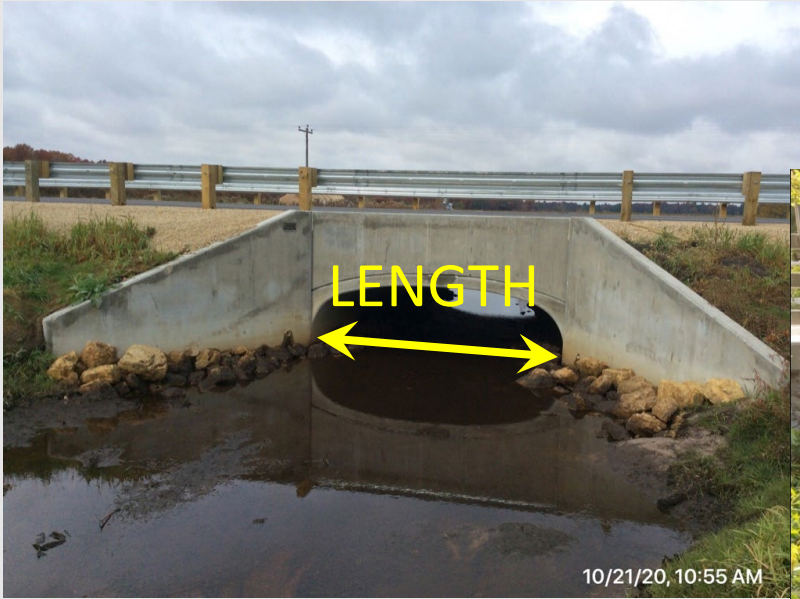
Precast Concrete Arch
