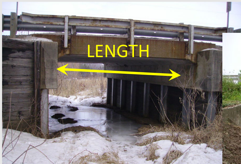
Concrete Flat Slab
