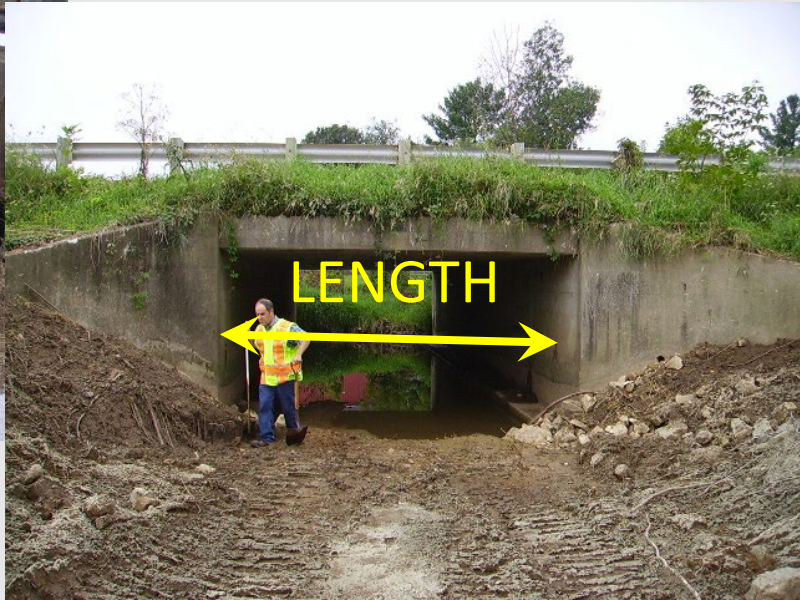
Buried Rigid Frame (no floor)
