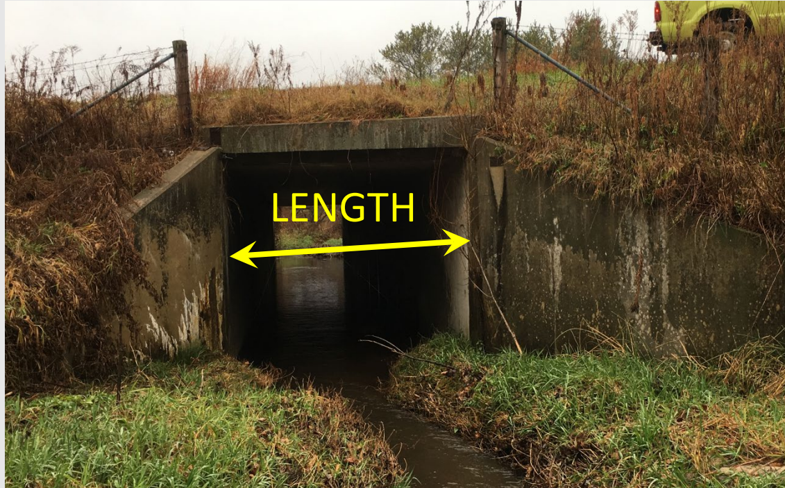
Single Concrete Box Culvert Pipe
