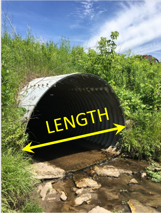
Steel Pipe Arch
