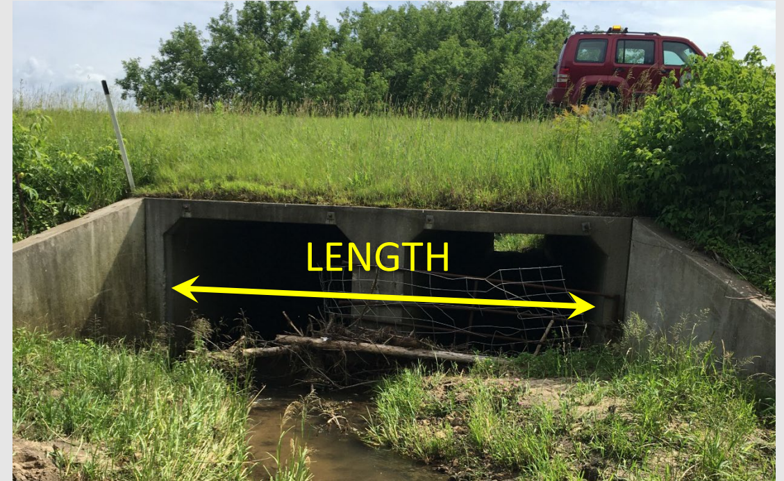
Double Barrel (multicell) Box Culvert
