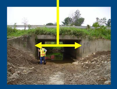
**Buried Concrete Rigid Frame** (no floor)
