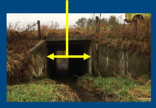
**Single-Cell Concrete Box Culvert**
