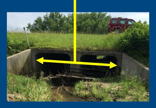
**Multi-Cell Concrete Box Culvert**
