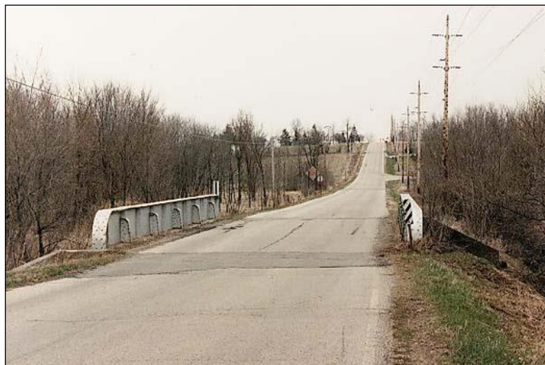
Figure 2.4.4.8-2: NSTM Through Girder Bridge.
