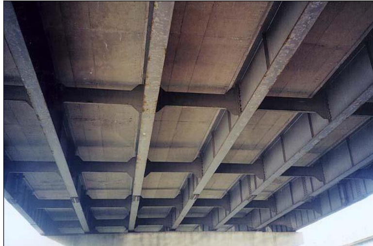
Figure 2.4.4-2: Steel Multi-Girder Bridge.
