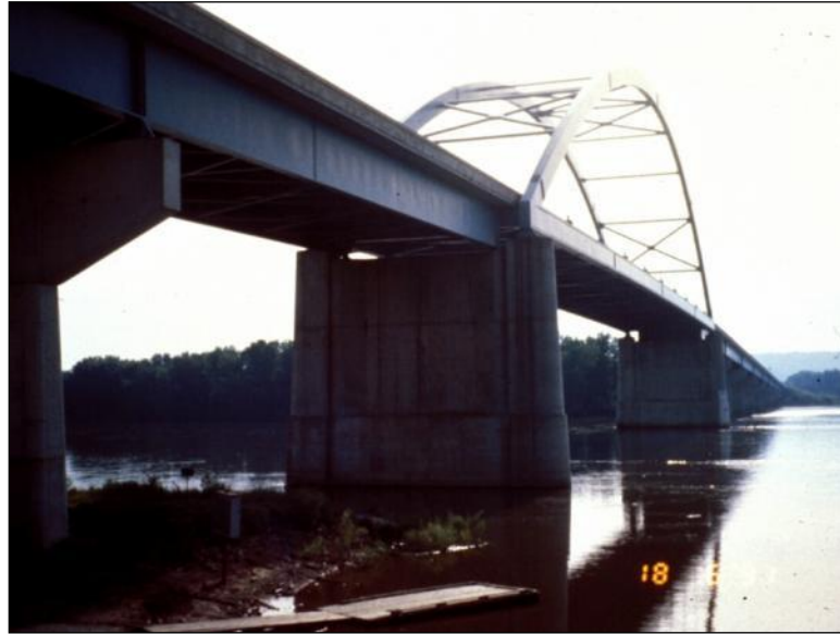
Figure 2.4.4-8: Steel Tied Arch Bridge.
