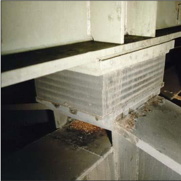
Figure 2.4.6.1-2: Elastomeric Bearing - Condition State 1.
