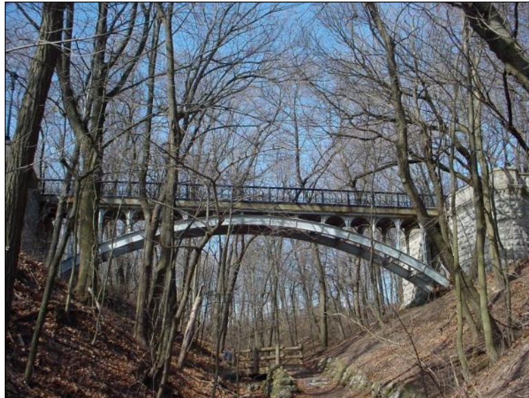
Figure 2.4.4-7: Steel Deck Arch Bridge.
