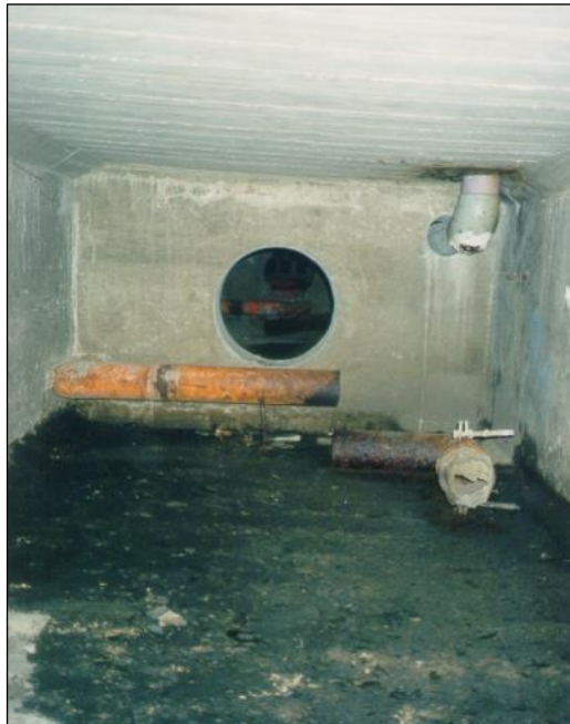
Figure 2.4.2.2-1: Inside of a Reinforced Concrete Box Girder.
