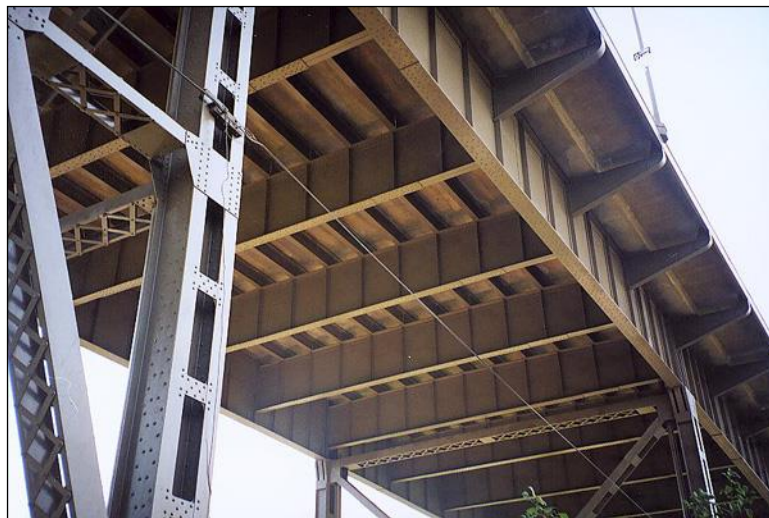
Figure 2.4.4.8-1: NSTM Two-Girder Bridge.
