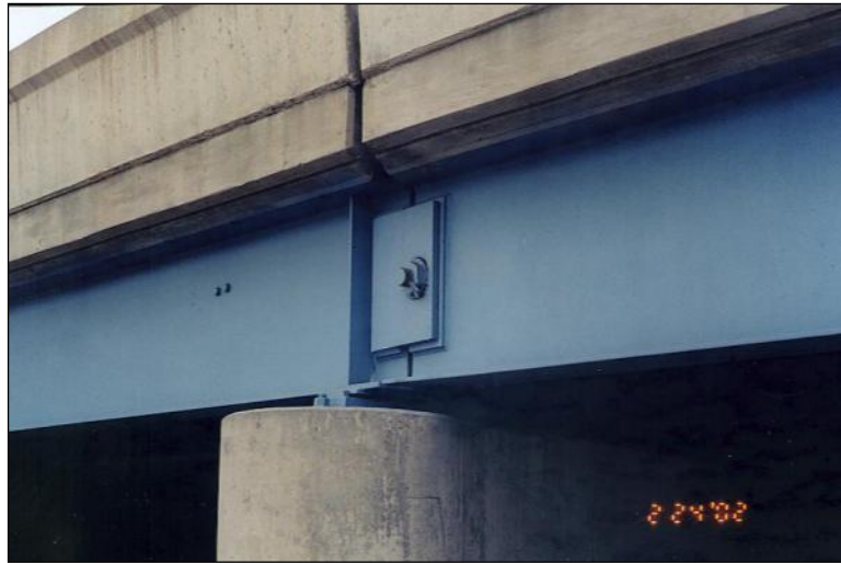
Figure 2.4.4.7-4: Steel Girders, Pin and Plate – Condition State 1.
