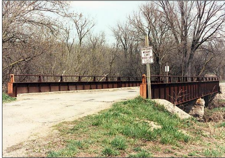
Figure 2.4.4-4: Steel Through Girder Bridge.
