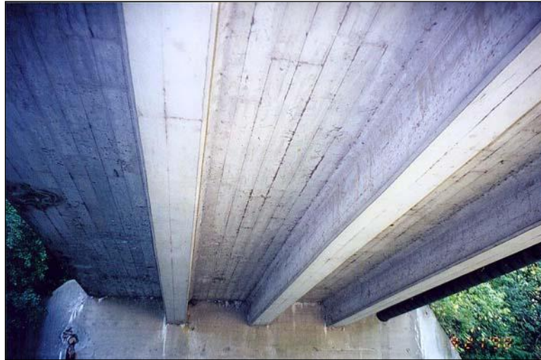
Figure 2.4.2.2-2: Reinforced Concrete Tee Beams – Condition State 1.
