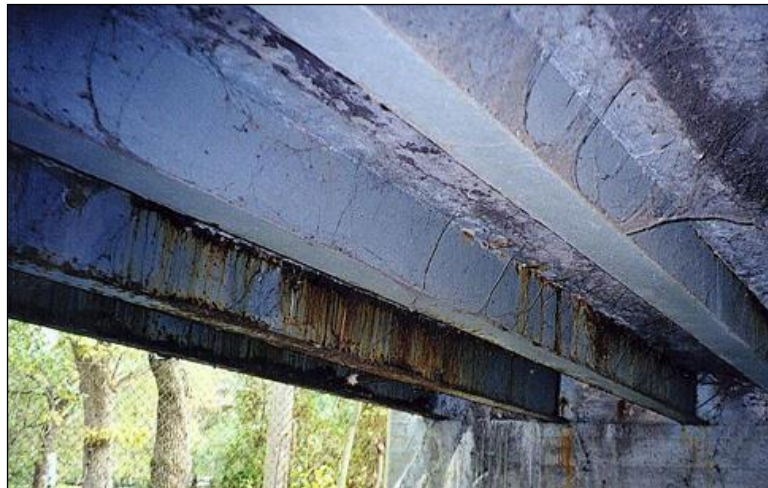
Figure 2.4.4-1: Rolled Steel Multi-beam Bridge.
