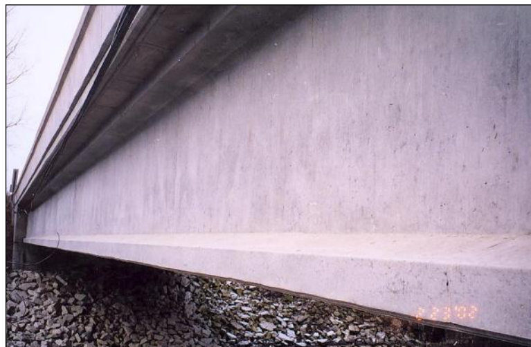
Figure 2.4.3.1-2: Prestressed I-Beam – Condition State 1.
