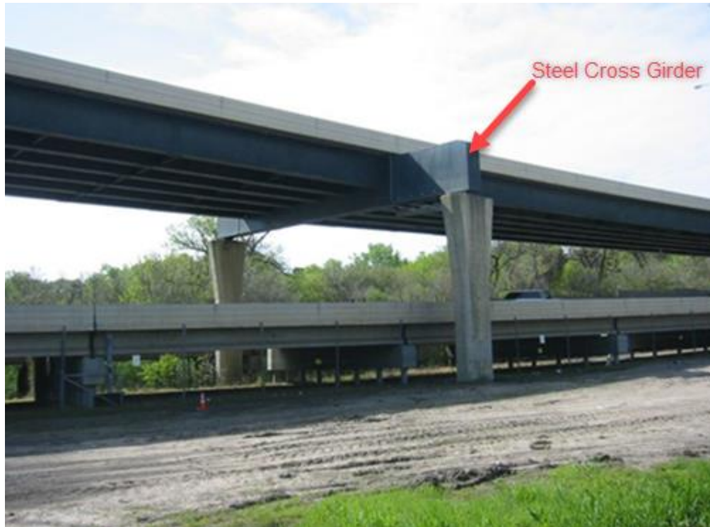
Figure 2.4.4.1-1: Steel Cross Girder – Closed Web/Box Girder
