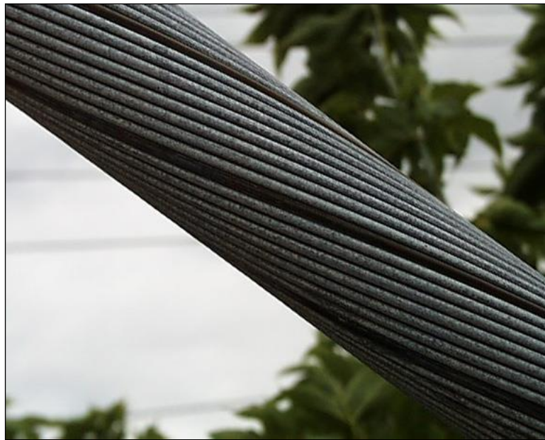
Figure 2.4.4.2-2: Galvanized Steel Cable – Condition State 1.
