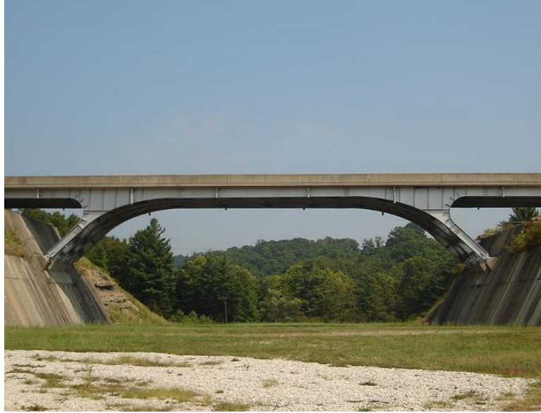
Figure 2.4.4-9: Steel Rigid Frame Bridge.
