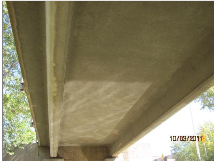
Figure 2.4.3-2: Double Tee Girder Bridge.
