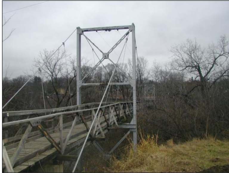
Figure 2.4.4-11: Steel Pedestrian Suspension Bridge.
