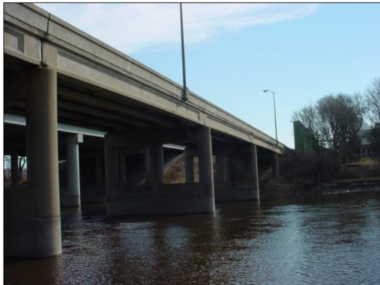
Figure 2.4.3.1-1: Prestressed Concrete I-Beam Bridge.
