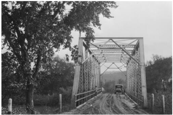
Heavier Vehicles on Older Bridges
