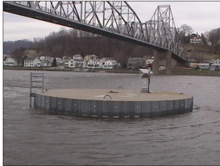
**Figure 2.9.2.1-1:** Cell Dolphin During Flood Conditions.
