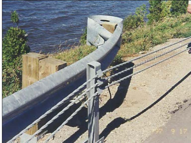
**Figure 2.9.3.1-1:** Section of Cable Guard Next to a Steel Plate Beam Guard.
