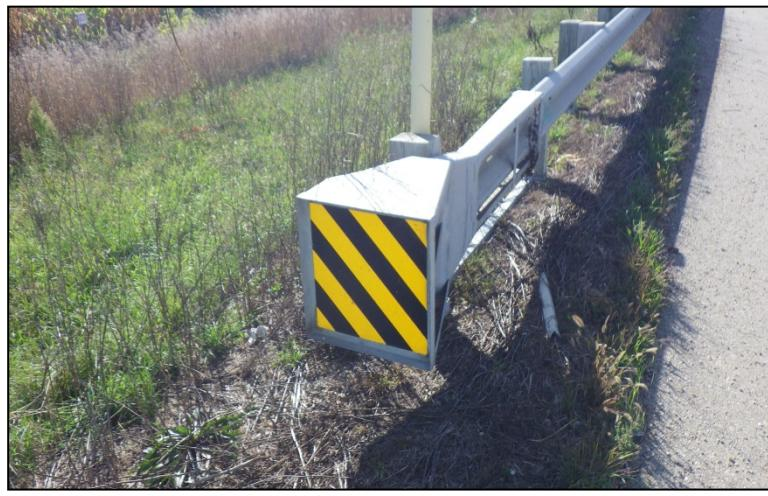
**Figure 2.9.3.2-1:** Newly Installed Beam Guard.
