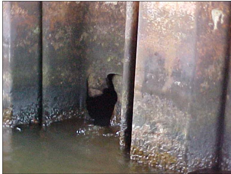
**Figure 2.9.4.1-1:** Cell Dolphin Deterioration.
