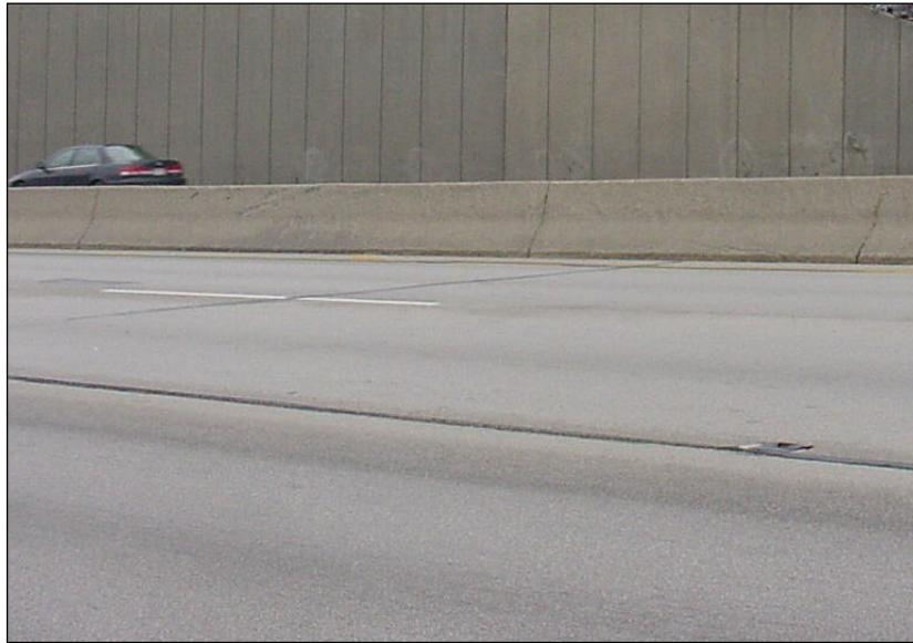
**Figure 2.9.5.4-1:** Concrete Median Barrier Wall.
