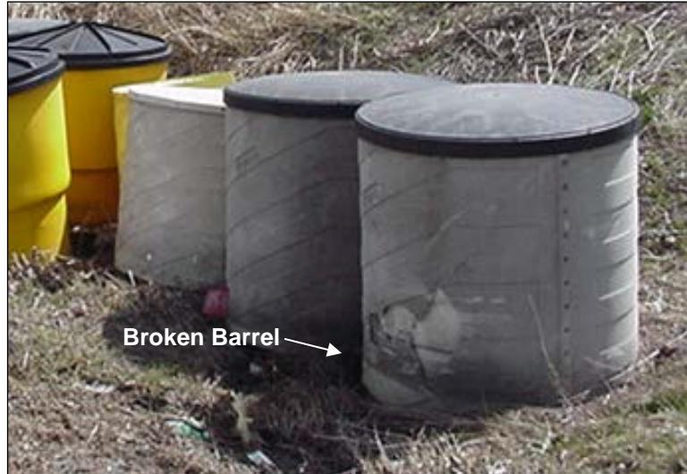
**Figure 2.9.5.3-1:** Damaged Impact Attenuator.
