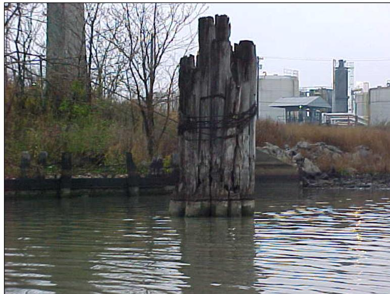
**Figure 2.9.4.2-1:** Pile Cluster Dolphin Deterioration.
