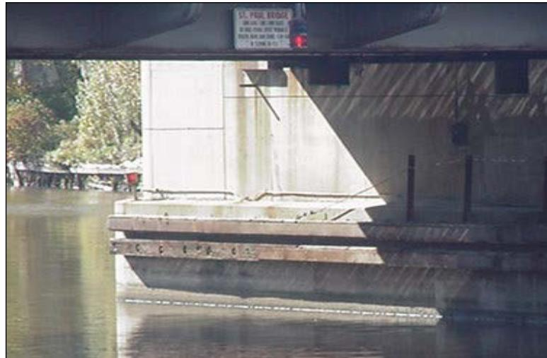
**Figure 2.9.2.3-2:** Substructure-Supported Timber Fender System.
