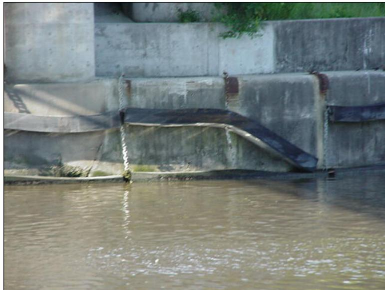
**Figure 2.9.4.3-1:** Failed Rubber Fender System.
