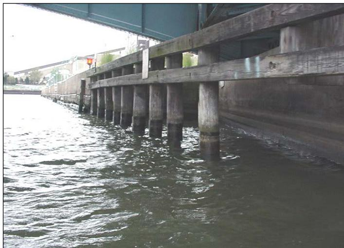
**Figure 2.9.2.3-1:** Independently Supported Timber Fender System.
