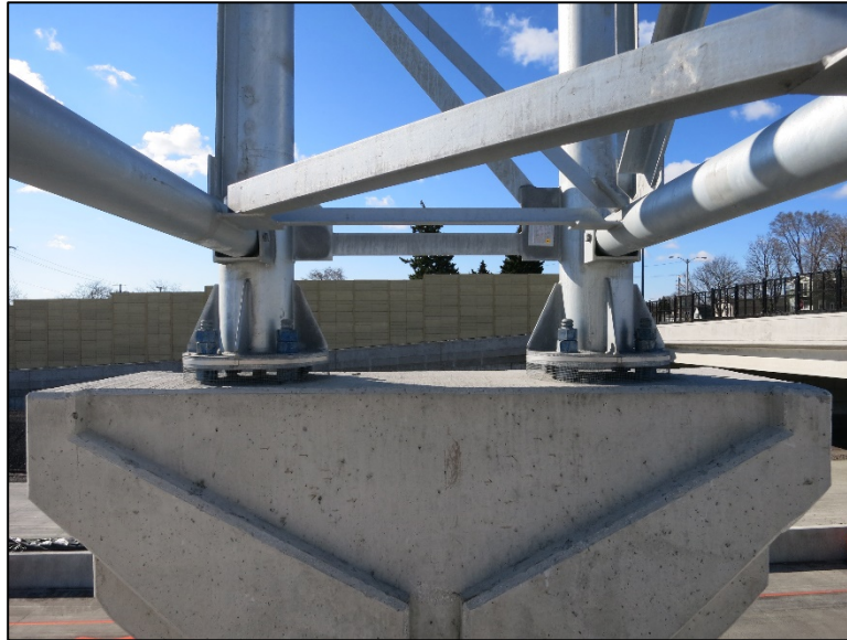
Figure 4.2.3-24: Four Chord Truss to Post Saddle Bracket Connection.
