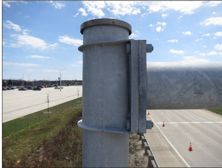
Figure 4.2.1-10: Typical Mast Arm Support Post Connection.
