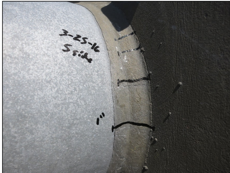
Figure 4.2.3-35: Transverse Weld Cracks Along Circumferential Socket Weld of Mast Arm to Vertical Plate Connection (Condition State 3)
