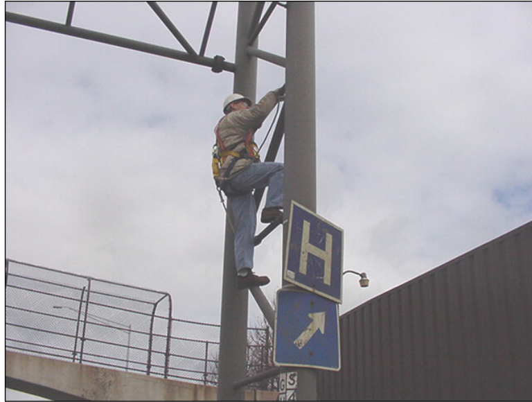
Figure 4.2.2-1: Inspector Climbing an End Support Frame.
