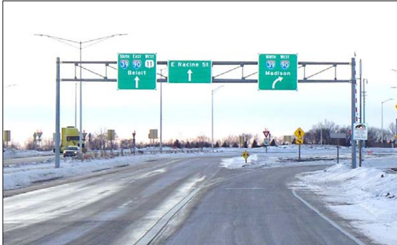
Figure 4.2.1-4: Typical Two-Chord Sign Support Structure.
