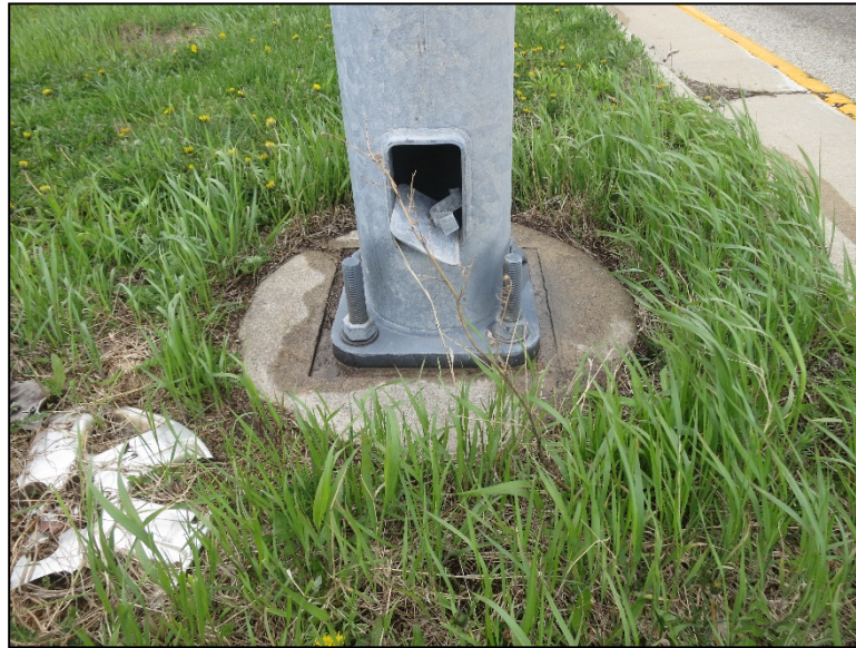
Figure 4.2.4-5: Handhole Cover Unsecured at Base of Signal Mast Arm Column (Condition State 3).
