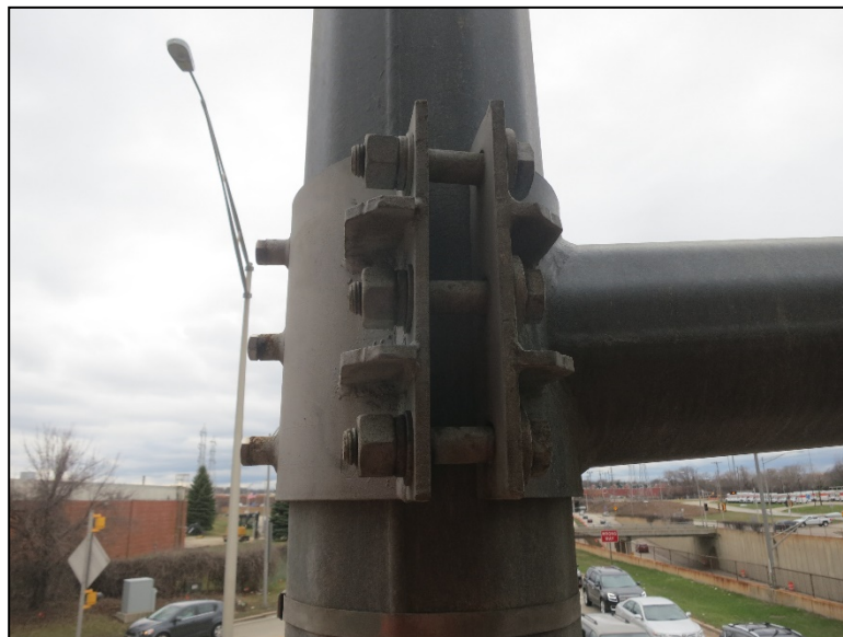
Figure 4.2.3-33: Column to Mast Arm Clamped Connection.
