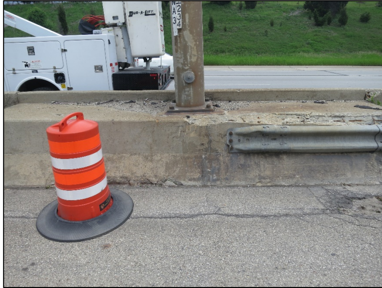
Figure 4.2.4-9: Deteriorated Barrier Wall with Approach Guardrail Protecting the Foundation of a Butterfly Sign Structure (CS 2)
