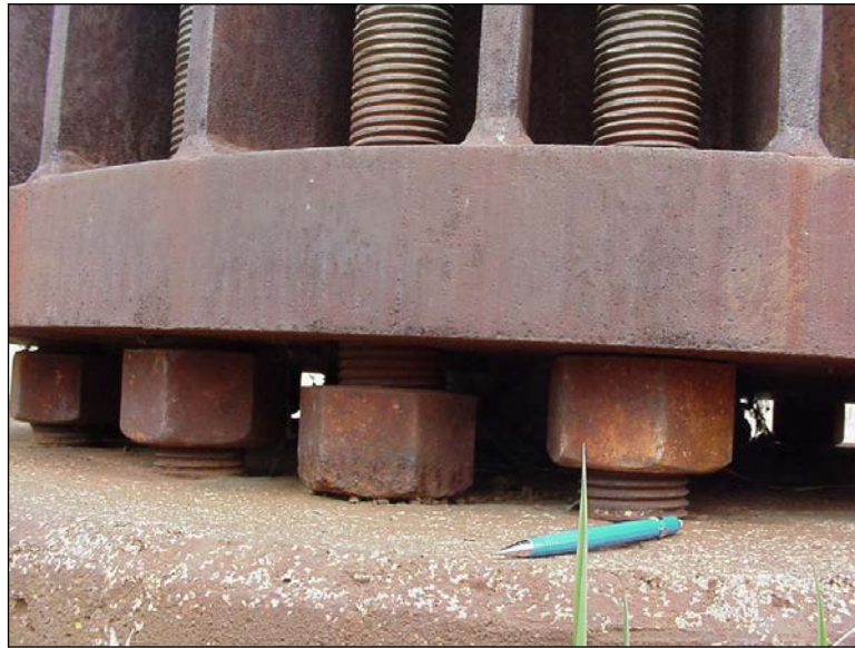
Figure 4.2.3-13: Leveling Nuts Not Fully In Contact with the Base Plate (Condition State 4).
