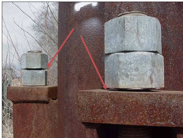
Figure 4.2.3-12: Anchor Nuts and Jam Nuts not Fully Tight to the Base Plate, or to Each Other (Condition State 4)
