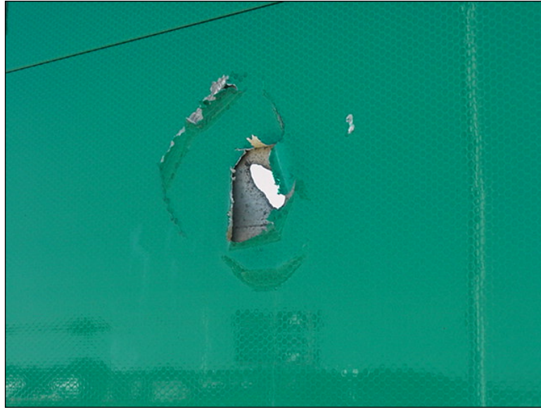
Figure 4.2.3-42: Damaged Sign Panel with Reflective Coating Beginning to Tear and Peel (Condition State 2)
