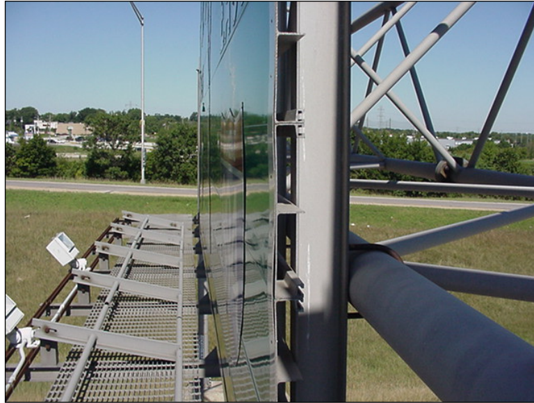
Figure 4.2.4-7: Catwalk with Handrails in Collapsed Position.
