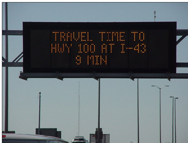
Figure 4.2.3-45: Typical Dynamic Message Sign.
