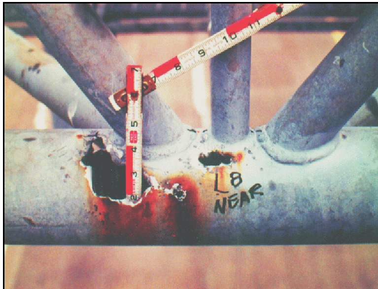
Figure 4.2.2-3: Corrosion in a Horizontal Steel Chord Member.
