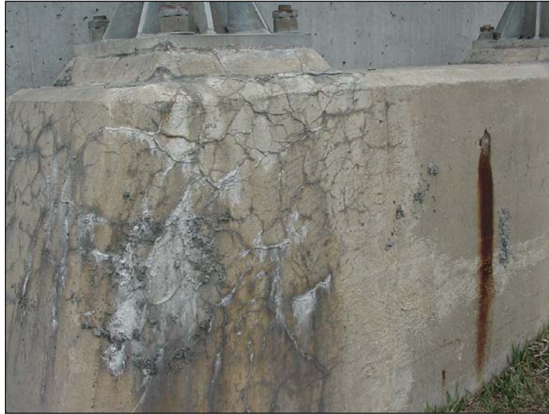
Figure 4.2.3-1: Map Cracking with Efflorescence on a Four Chord Sign Structure (Condition State 3).
