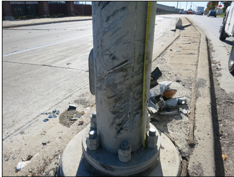
Figure 4.2.4-13: Scraped Galvanized Coating at Base of Column Due to Impact. Bare Steel Exposed in Several Locations (Condition State 3).
