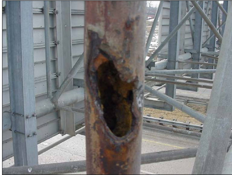
Figure 4.2.2-2: Steel Corrosion in a Vertical Member.
