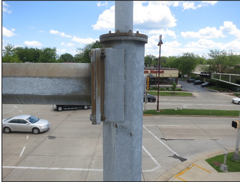
Figure 4.2.3-53: Signal Mast Arm with Luminaire Post Anchored to Top of Post. All of Luminaire is Inspected Under Element 8711.
