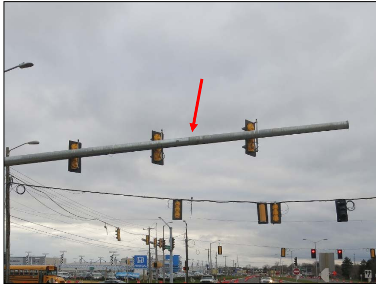
Figure 4.2.3-38: Slip Joint Extending Length of Mast Arm.
