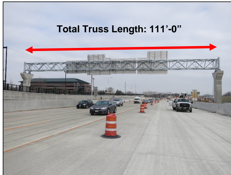
Figure 4.2.3-19: Four Chord Truss.
