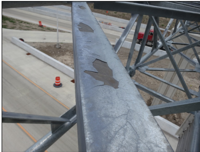
Figure 4.2.4-12: Cracked, Chipped and Peeling Galvanized Protective Coating on a Four-Chord Upper Diagonal Member (Condition State 3)
