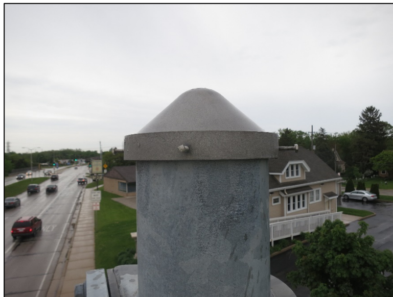
Figure 4.2.4-6: Column Cap for a Two-Chord Sign Structure.
