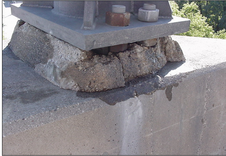
Figure 4.2.3-7: Deteriorated Grout Pad (Condition State 3).
