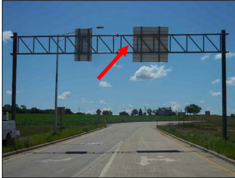
Figure 4.2.2-8: Right Truss Installed Upside Down. Truss Diagonals Should Run Down Towards Center From Upper Chord.
