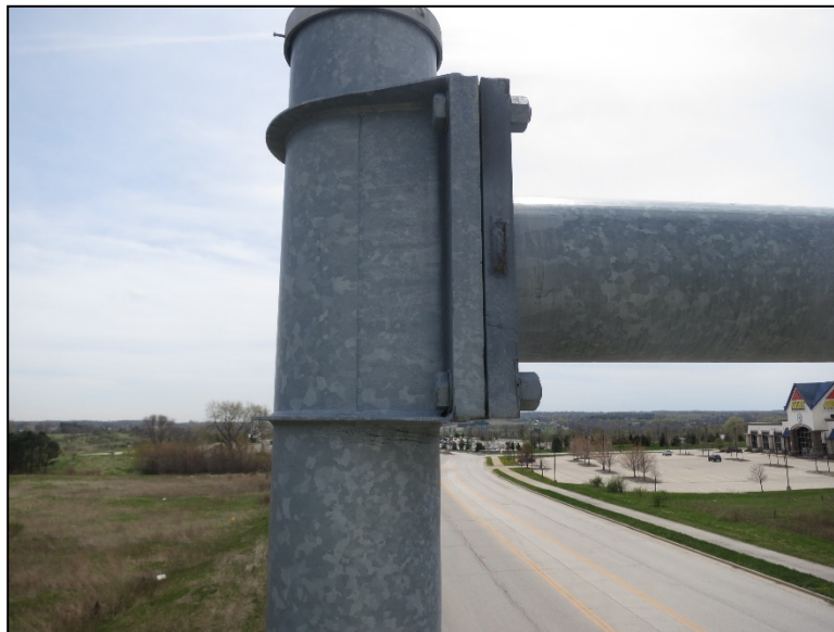
Figure 4.2.3-31: Column to Arm Connection with Horizontal Column Plates Welded to Vertical Plate. Note Washers Improperly Included Between Plates.
