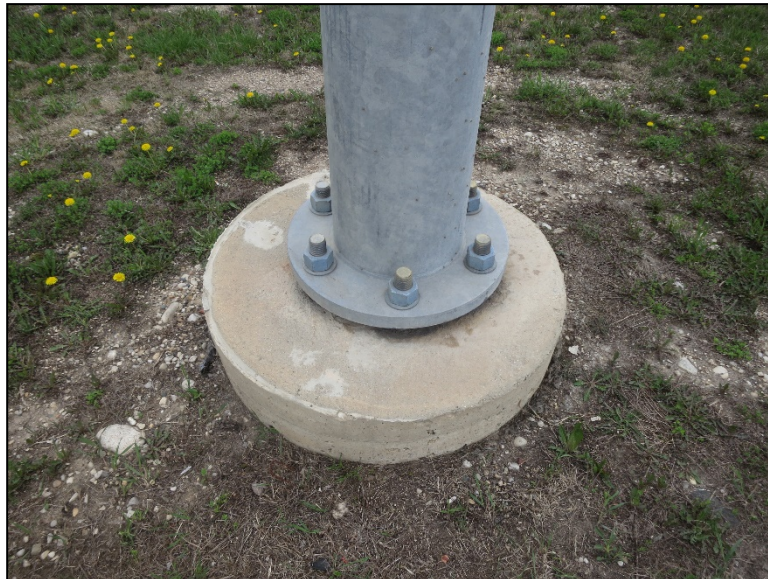
Figure 4.2.3-6: Anchor Rods Installed Offset from Center Foundation (Condition State 2 if Verified by Engineer within Report).
