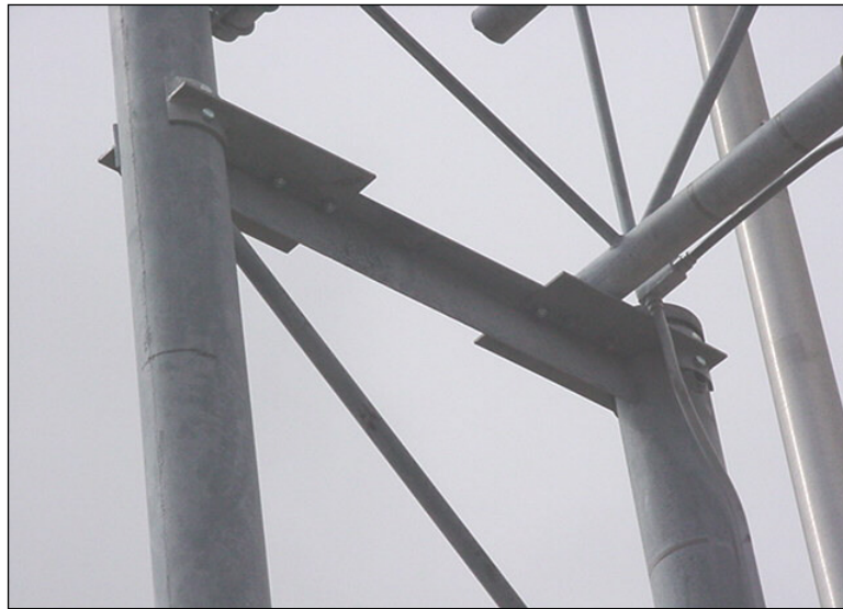
Figure 4.2.3-27: Tri-Chord Bolted T-Section Repair.
