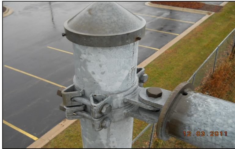
Figure 4.2.3-29: Typical Monotube Chord to Support Column Connection.
