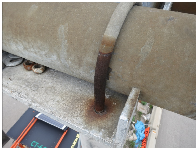
Figure 4.2.3-30: Corroded U-Bolt Connection Securing Horizontal Sign Support Member to the Post of a Butterfly Sign Structure (Condition State 2).
