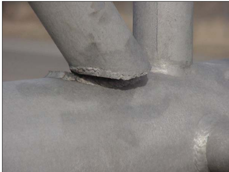
Figure 4.2.2-5: Broken Weld at an Aluminum Diagonal Member.
