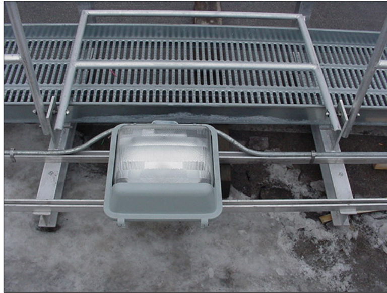
Figure 4.2.4-3: Typical Sign Structure Luminaire.
