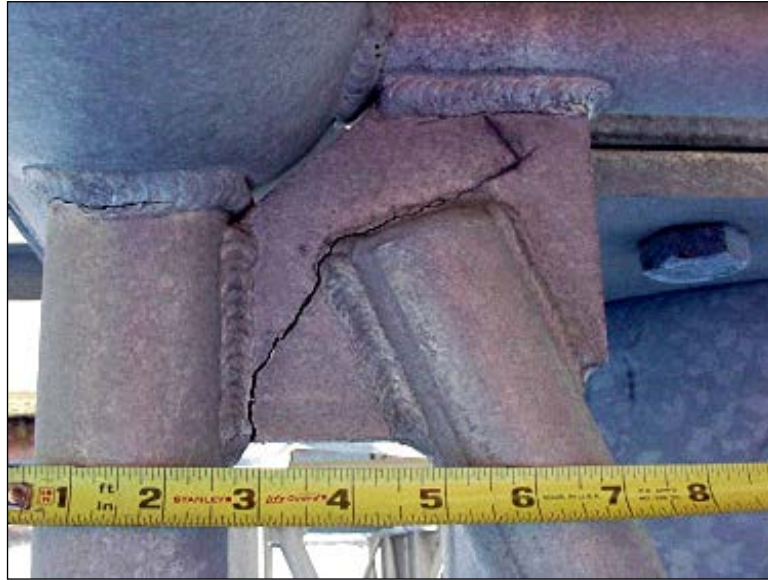
Figure 4.2.2-6: Crack through an Aluminum Gusset Plate.
