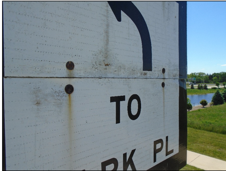
Figure 4.2.3-44: Sign Surface Cracked and Fading (Condition State 3)
