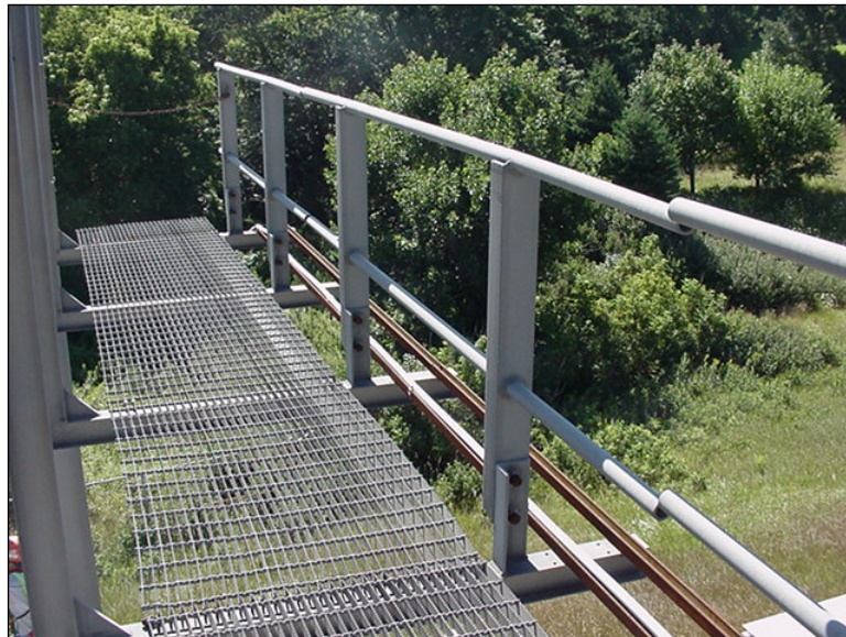
Figure 4.2.4-8: Catwalk with Handrails in Upright Position.
