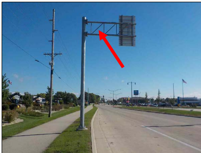
Figure 4.2.2-7: Truss installed upside down. Diagonals of Cantilever Should Angle Down Towards Sign Panel.
