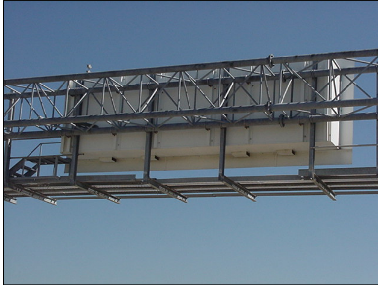
Figure 4.2.3-46: Typical Dynamic Message Sign, Rear View.
