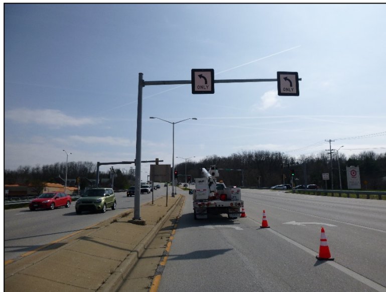
Figure 4.2.1-9: Typical Mast Arm Sign Support.
