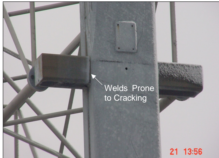
Figure 4.2.3-25: Square Stubs Welded to Support Column.
