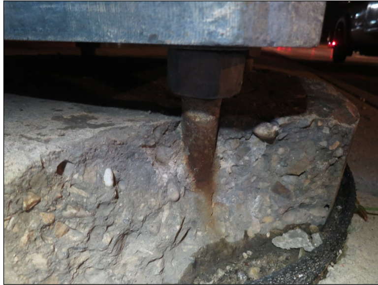
Figure 4.2.3-5: Foundation Spall Exposing Anchor Rod (Condition State 3).
