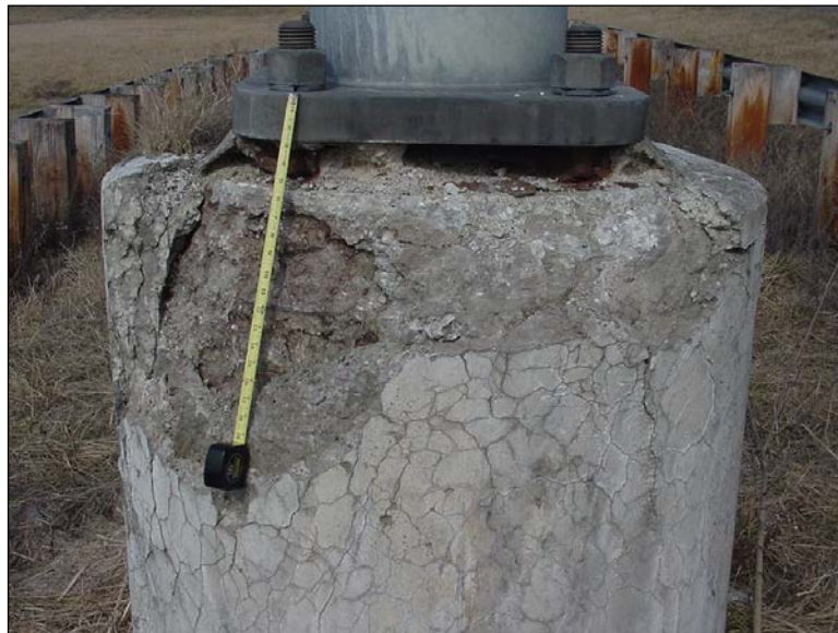
Figure 4.2.3-2: Map Cracking with Delamination and Spall on a Butterfly Foundation (Condition State 3).
