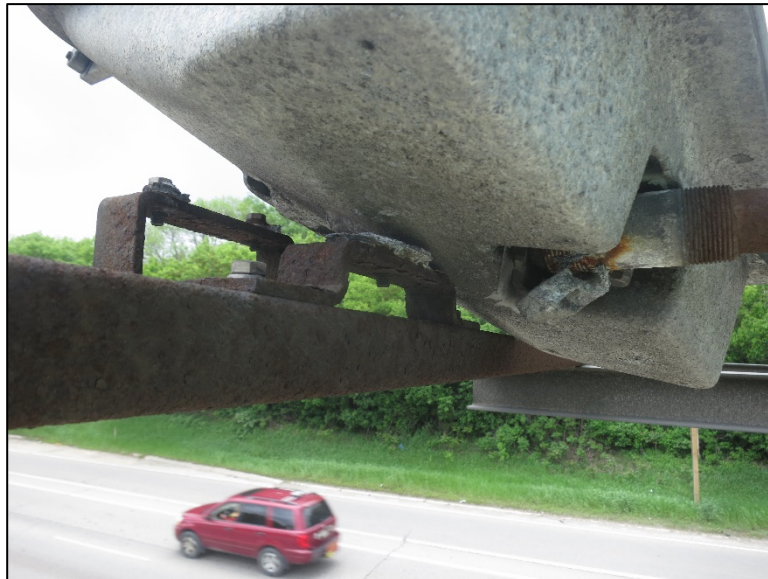
Figure 4.2.4-4: Failed Connections of a Luminaire to U-Bracket on a Butterfly Sign Structure (Condition State 4)
