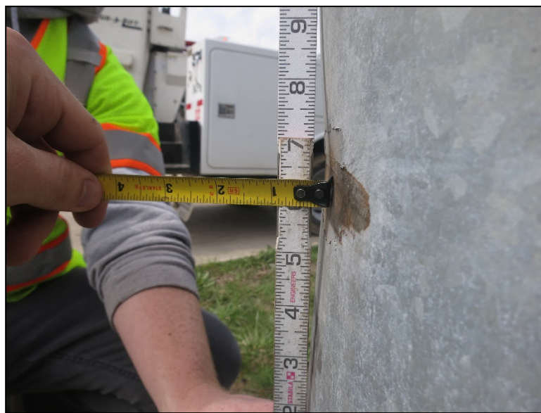
Figure 4.2.3-18: Base of Post Distorted Out of Plane Due to Impact (Condition State 3).
