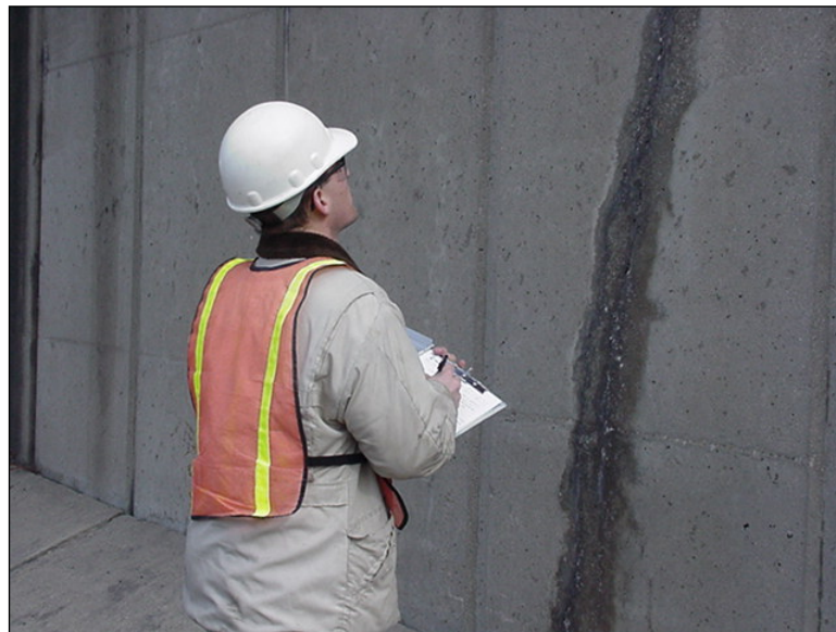
Figure 5.2.1-1: Inspector Conducting Visual Inspection.
