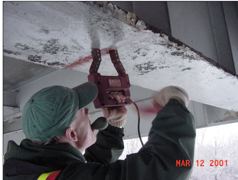
Figure 5.7.2-1: MT on a Built-Up Plate Bridge Girder Butt-Weld.
