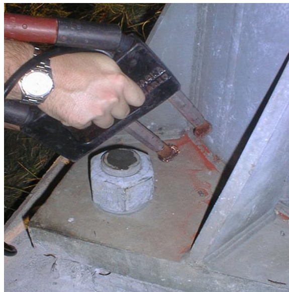
Figure 5.7.2-2: MT on a Sign Structure Base.
