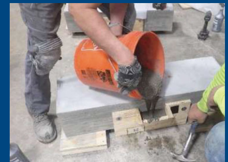
Draft Report: Form-and-pour in overhead orientation
