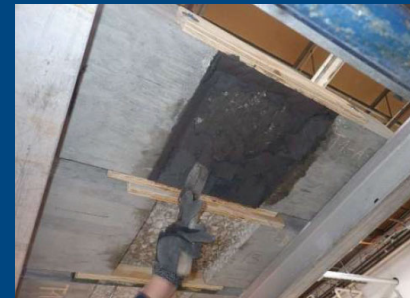
Draft Report: Hand-applied patch in overhead orientation
