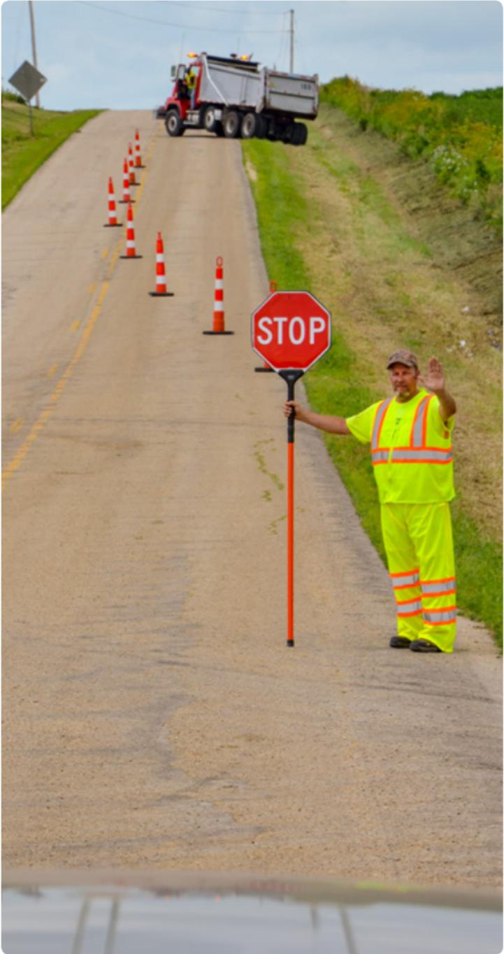
Figure 3: Stopping first vehicle from shoulder
