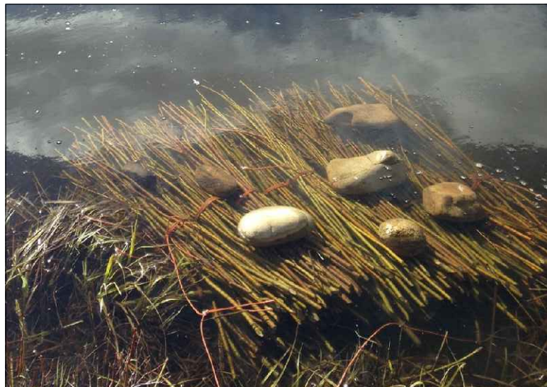
COMPLETELY SUBMERGED WILLOW STAKES
