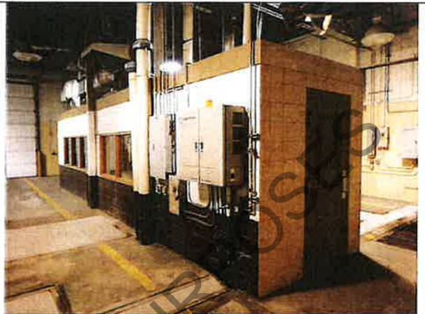
View of Concrete Block Structure Separating Bays
