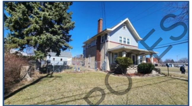
West Elevation of Residence
