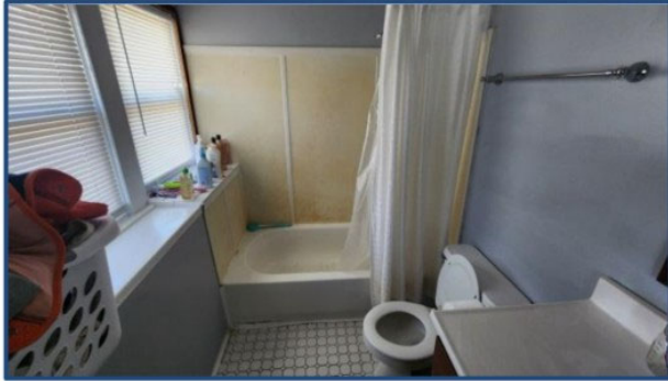
Second Floor Full-Bathroom (View 1)
