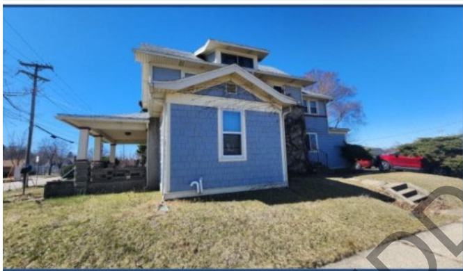
East Elevation of Residence
