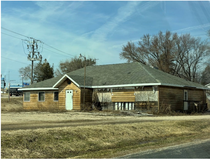
Front of building
