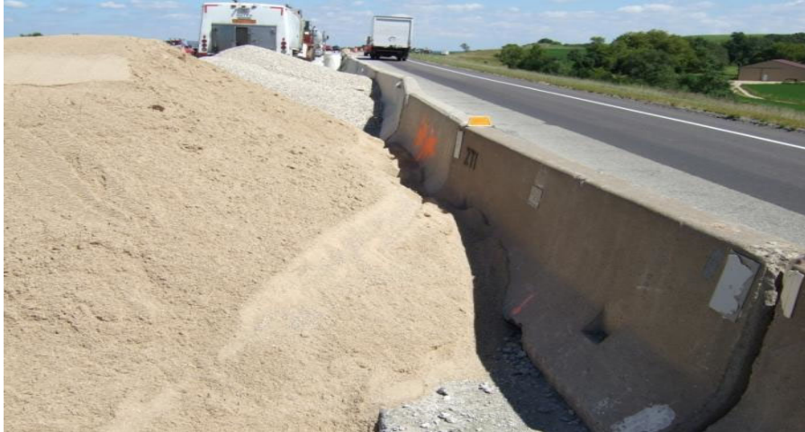
FIGURE 145-21 Insufficient Clearance Behind Temporary Barrier
