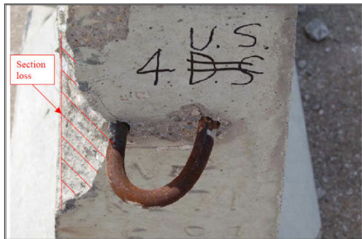
FIGURE 145-5 Loop Out of Alignment
