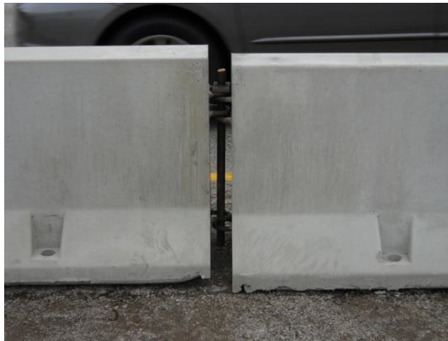
FIGURE 145-22 Improper Connection of 12.5' Temporary Barrier
