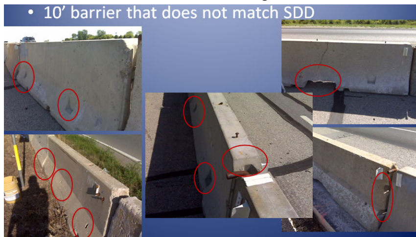
FIGURE 145-23 Barrier Not Matching Standard Details
