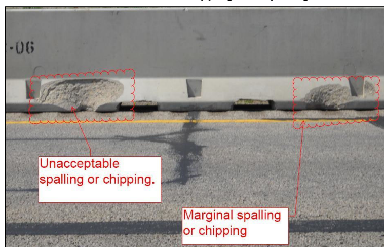
FIGURE 145-15 Chipping and Spalling
