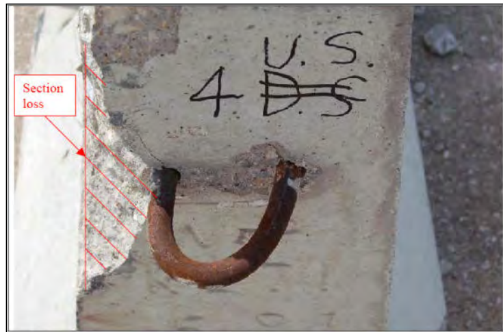
FIGURE 145-5 Loop Out of Alignment
