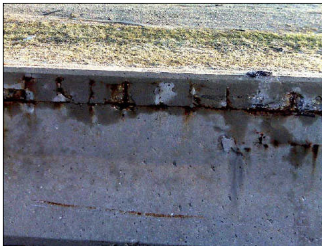
FIGURE 145-10 Exposed Steel Reinforcement
