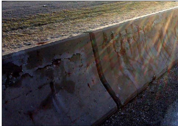
FIGURE 145-11 Exposed Steel Reinforcement
