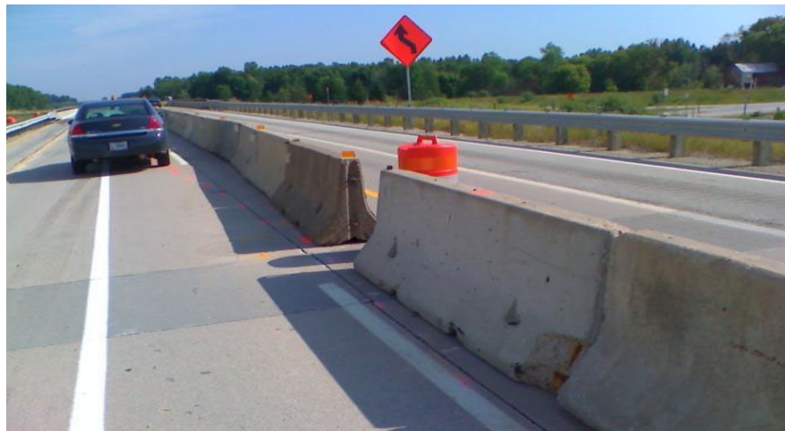
FIGURE 145-20 Gap in Barrier
