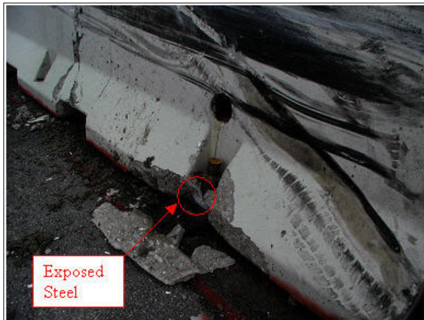
FIGURE 145-8 Anchor Hole Damage
